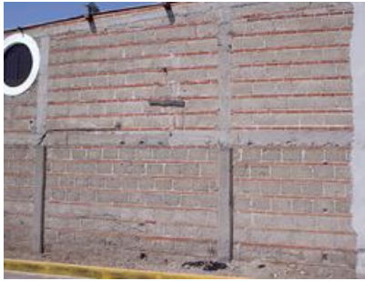
Figure 8. Combined and confined masonry house: 1 course of bricks alternate with 1 course of concrete blocks.
