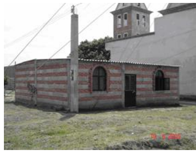
Figure 9. One-story combined and confined masonry house: 3 courses of bricks alternate with 1 course of concrete blocks.
