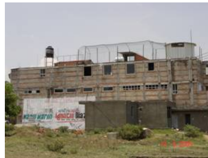
Figure 4. Three-story combined and confined masonry apartment building: 3 courses of bricks alternate with 2 courses of concrete blocks.
