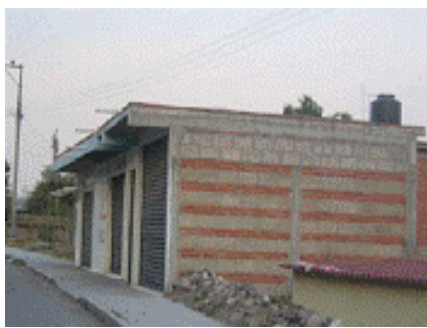
Figure 6. Combined and confined masonry store: 2 courses of bricks alternate with 1 course of concrete blocks.
