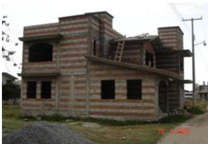
Figure 1. Most common configuration of combined and confined masonry: Figure 2. States in Central Mexico where combined and confined masonry
