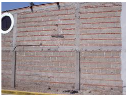
Figure 8. Combined and confined masonry house: 1 course of bricks alternate with 1 course of concrete blocks.
