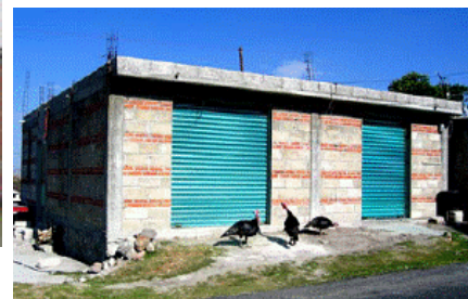
Figure 7. Combined and confined masonry store: 2 courses of bricks alternate with 2 courses of concrete blocks.
