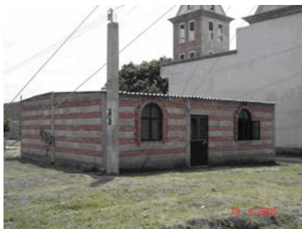
Figure 9. One-story combined and confined masonry house: 3 courses of bricks alternate with 1 course of concrete blocks.
