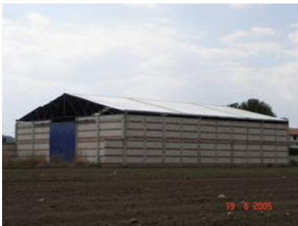
Figure 3. Combined and confined masonry warehouse: 3 courses of bricks alternate with 3 courses of concrete blocks.
