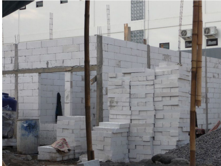
Figure 3. Building regulations need to specify safe yet practical ways of using new materials, such as these light-weight blocks.
