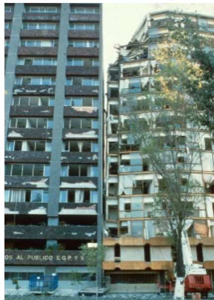
Figure 2. Two buildings have pounded each other with one far more seriously damaged than the other.
