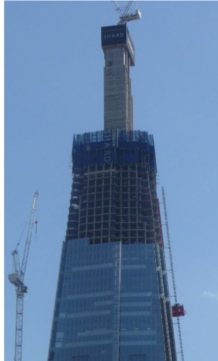
Figure 3. An example of a reinforced concrete core in a building under construction.
