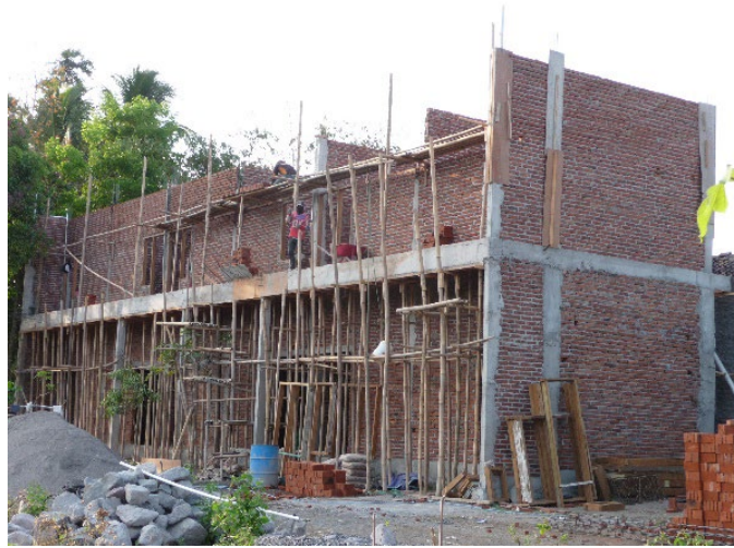
Figure 2. A confined masonry house under construction.
