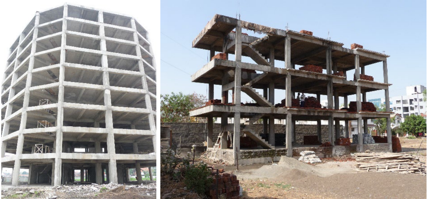
Figure 1. These two buildings resist earthquakes through the strength of their columns and beams. Walls and cladding are yet to be constructed.
