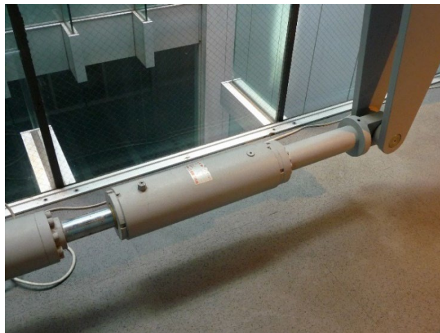
Figure 3. A damper to reduce earthquake movements.
