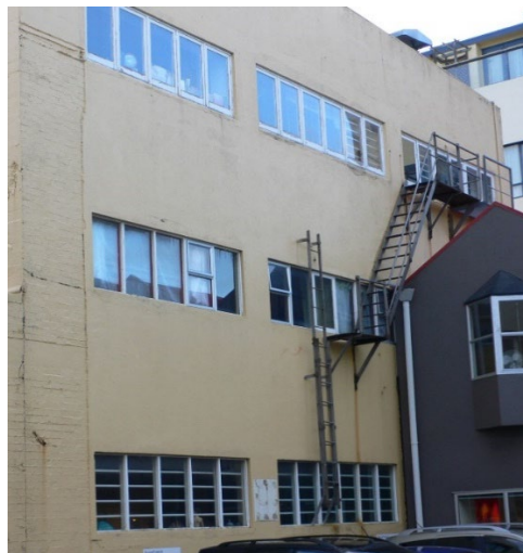
Figure 2. Normal height columns have been shortened from the perspective of resisting horizontal forces by partial-height infill walls.
