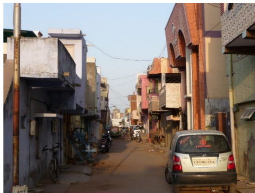
Figure 2. Buildings with off-set infill walls line this street.
