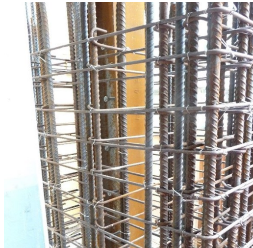
Figure 3. Column reinforcement is visible before the concrete is cast. The reinforcement consists of vertical bars that resist bending, and horizontal ties that stop the column concrete from disintegrating and dislodging.
