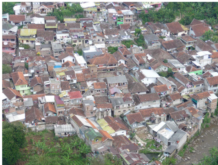
Figure 2. Codes and their implementation are necessary to improve the earthquake-safety of this type of housing.
