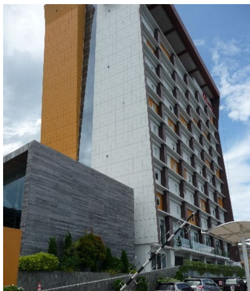
Figure 3. The base-isolated Ibis Hotel, Padang, Indonesia.
