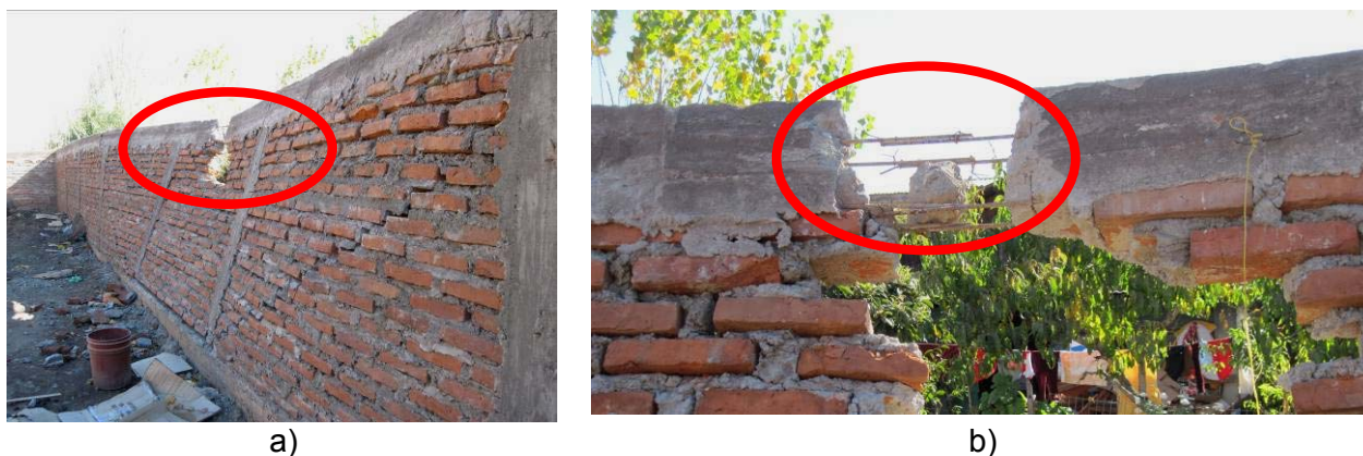
Figure 17. Collapse of a confined masonry fence in the 2010 Maule, Chile earthquake due to out-of-plane seismic effects: a) collapsed fence showing the RC tie-beam failure, and b) detail of RC tie-beam showing excessively short lap splice length in the longitudinal reinforcement (M. Astroza).
