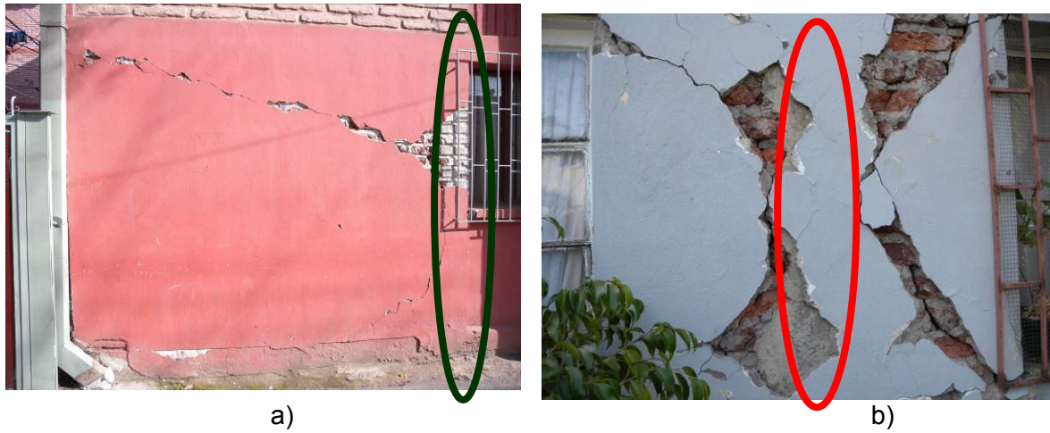
Figure 27. In-plane shear cracking of piers in confined masonry walls: a) a confined masonry panel with RC tie-columns at both ends (note RC tie-column highlighted with a black ellipse), and b) unconfined opening (note RC tie-column at the middle of the pier highlighted with a red ellipse) (Brzev et al., 2010).
