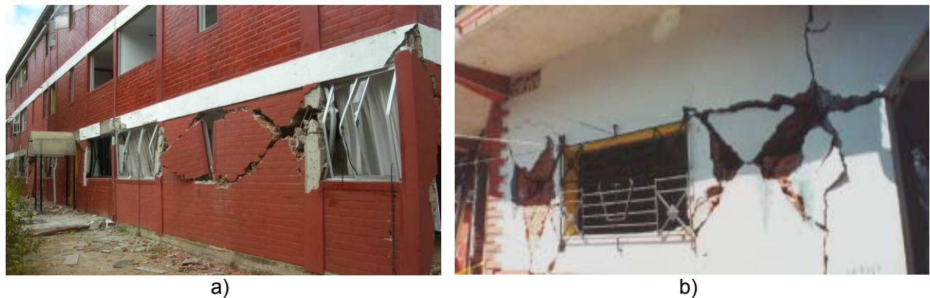
Figure 12. In-plane shear failure of poorly confined masonry walls: a) the 2010 Maule, Chile earthquake (M. Astroza), and b) the 2001 El Salvador earthquake (EERI, 2001).
