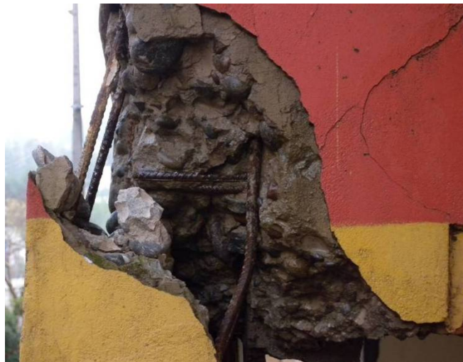
Figure 23. Buckling of longitudinal reinforcement due to inadequate confinement in the end zones of RC tie-columns (Brzev et al., 2010).
