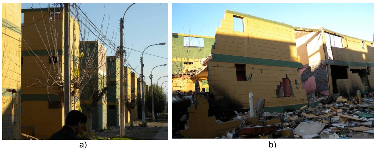
Figure 19. Collapse of a three-story confined masonry building in Santa Cruz, Chile due to the February 2010 Maule earthquake: a) building complex, and b) a building that experienced collapse at the ground floor level (S. Brzev).
