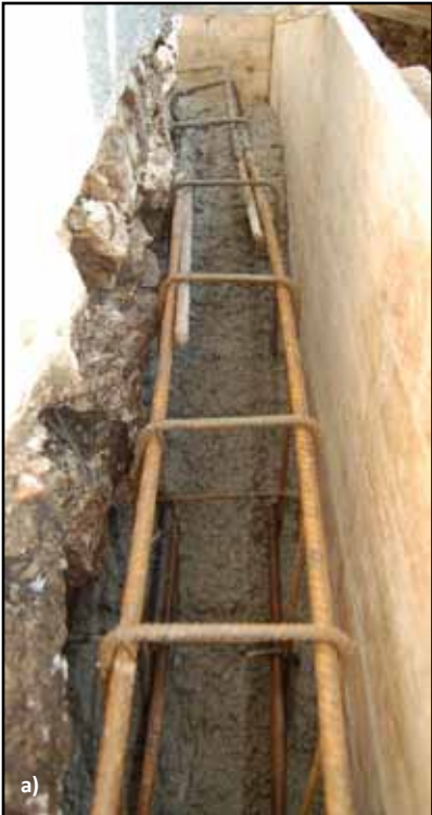
Figure 4.30 Strengthening a stone masonry foundation: a) reinforcement cage and formwork, and b) new reinforced concrete foundation under construction (photos: M. Lutman)
