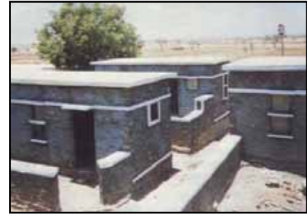
Figure 3.15 Stone masonry houses with RC lintel bands built after the 1993 Maharashtra, India, earthquake (source: GOM 1998)
