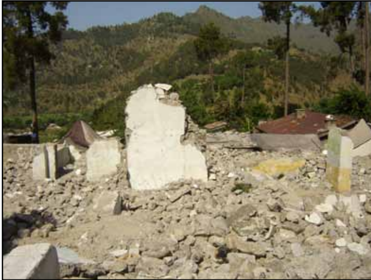
Figure 2.3 Collapse of stone masonry buildings, 2009 Bhutan earthquake (photo: K. Vatsa)
