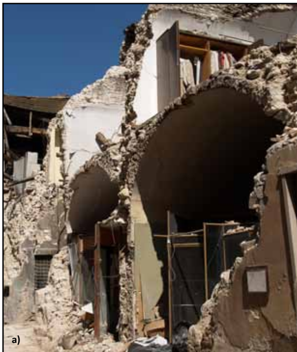
Figure 1.9 Vaults in stone masonry buildings in Italy: a) and b) stone masonry vaults in L'Aquila (photos: T. Schacher) and c) an example of a brick vault from Pavia (photo: S. Brzev)
