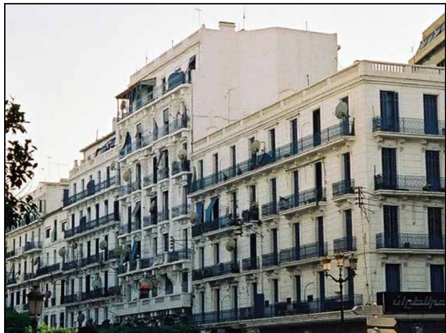
Figure 1.4 Six-story stone masonry building in Algiers, Algeria (photo: S. Brzev)
