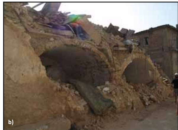
Figure 1.9 Vaults in stone masonry buildings in Italy: a) and b) stone masonry vaults in L'Aquila (photos: T. Schacher) and c) an example of a brick vault from Pavia (photo: S. Brzev)
