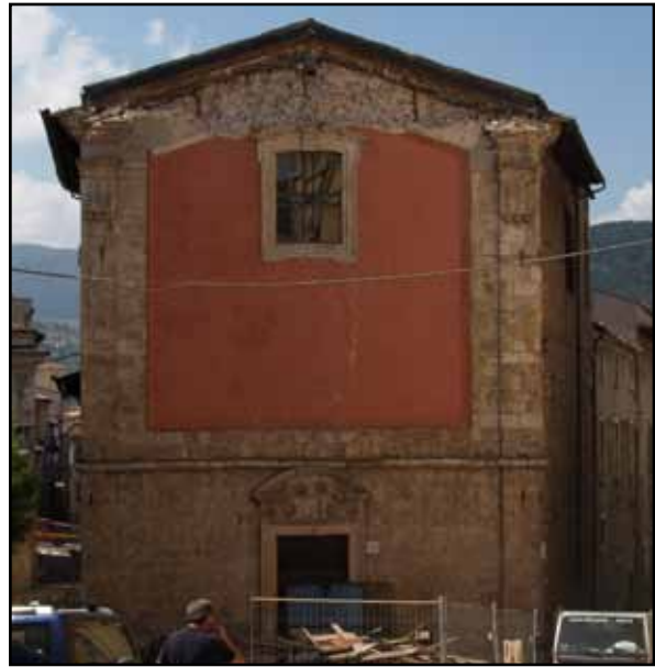
Figure 2.16 A building with roof-to-wall anchors survived the 2009 L'Aquila, Italy, earthquake (photos: T. Schacher)
