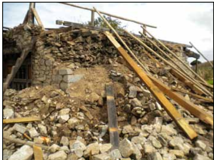
Figure 2.4 Collapsed stone masonry buildings, 2009 Bhutan earthquake (photo: K. Vatsa)
