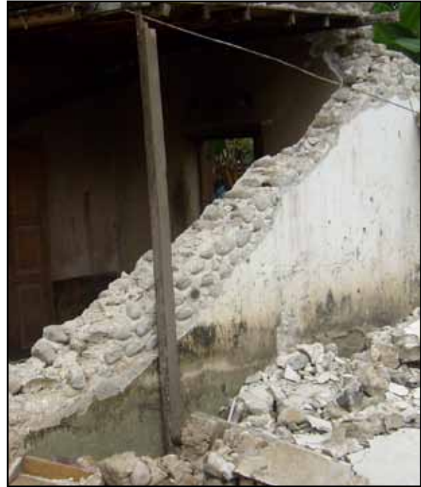
Figure 1.19 Round stone boulders used for traditional stone masonry construction in Padang, Indonesia (photo: J. Bothara)
