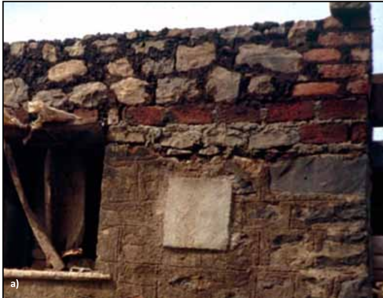
Figure 4.6 An example of a field application of an RC band in an existing stone masonry building in Maharashtra, India: a) RC band installation completed (note brick edging at the band level and a newly constructed portion of the wall above the band), and b) RC band at the roof level underneath the timber beams (note that roof is supported by an interior timber frame) (photos: S. Brzev)
