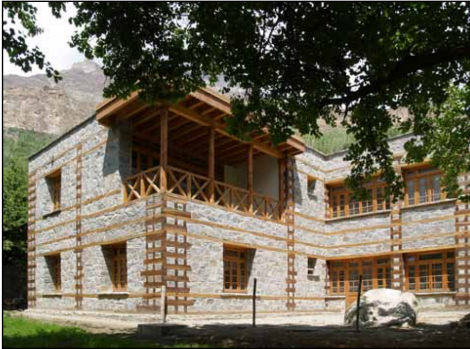
Figure 1.29 Stone masonry construction with timber bands in Pakistan (photo: T. Schacher)
