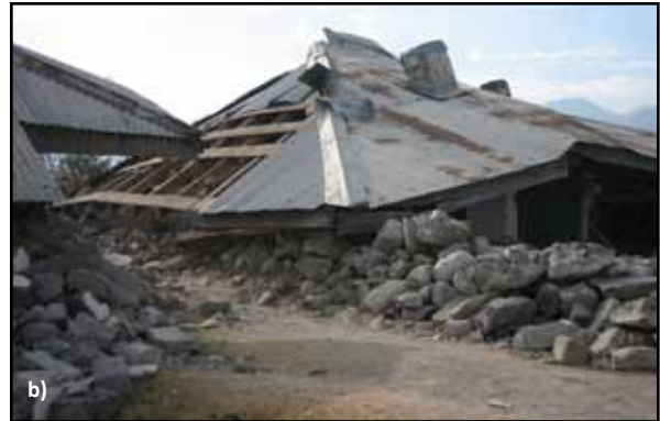
Figure 2.18 Collapse of roof structures due to the loss of gravity load-bearing capacity of stone walls in the 2005 Kashmir, Pakistan, earthquake: a) reinforced concrete roof, and b) timber and steel roof (photos: M. Tomazevic)
