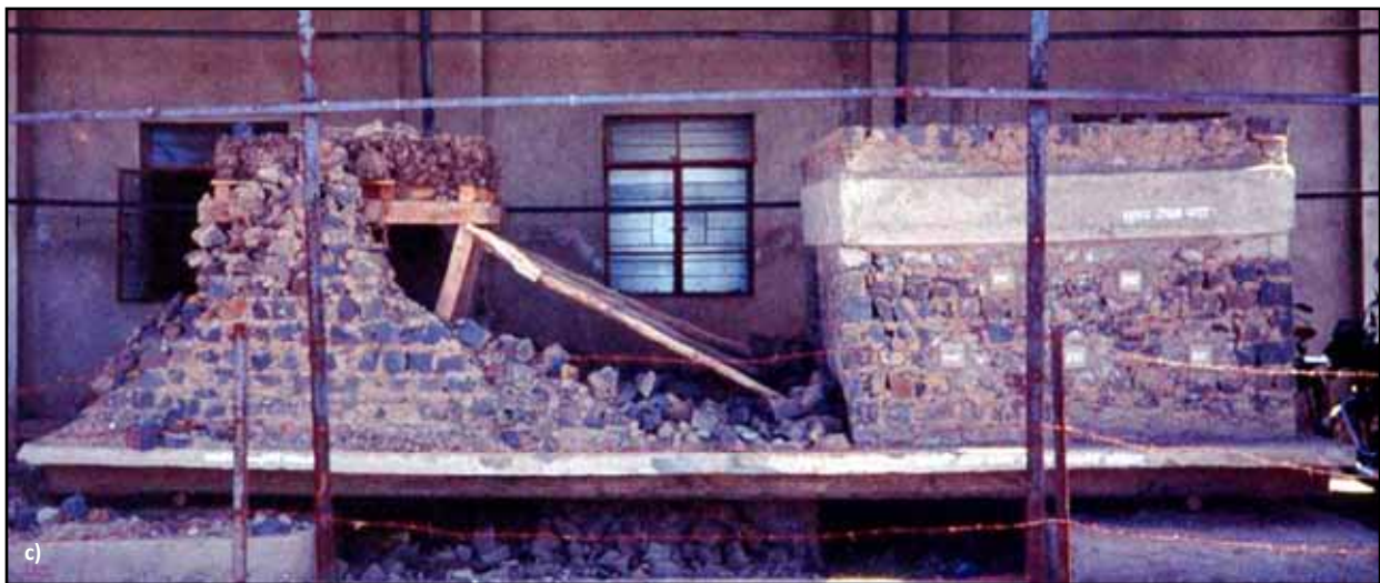
Figure 4.1 Effectiveness of seismic retrofitting methodology for stone masonry buildings: a) strengthened model, b) unstrengthened model after testing, and c) models at the end of the experiment (unstrengthened model shown on the left) (source: GOM 1998)
