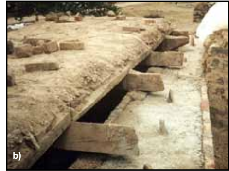
Figure 4.6 An example of a field application of an RC band in an existing stone masonry building in Maharashtra, India: a) RC band installation completed (note brick edging at the band level and a newly constructed portion of the wall above the band), and b) RC band at the roof level underneath the timber beams (note that roof is supported by an interior timber frame) (photos: S. Brzev)
