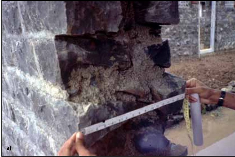
Figure 3.27 Stone masonry in cement mortar with a wall thickness limited to 450 mm (note through-stones) (photos: S. Brzev)
