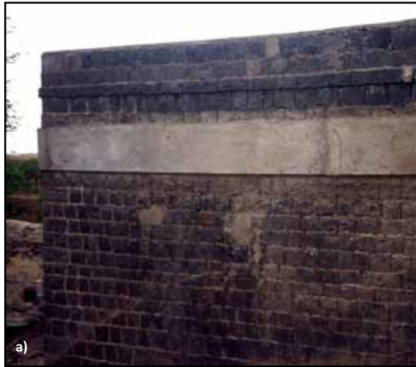
Figure 4.8 Construction of a reinforced concrete bandage: a) a retrofit application in Maharashtra, India and b) concept (source: GOM 1998)
