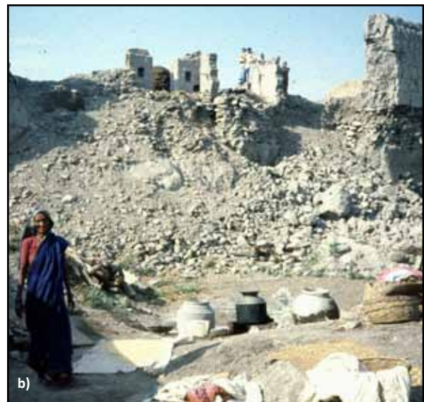
Figure 2.2 Extensive damage to stone masonry buildings in Indian earthquakes: a) the 2001 Bhuj, Gujarat, earthquake (photo: C.V.R. Murty), and b) the 1993 Maharashtra earthquake (photo: S. Brzev)
