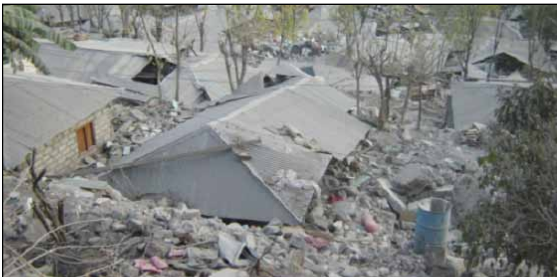
Figure 2.17 Collapse of stone masonry buildings with hipped roofs in the 2005 Kashmir, Pakistan, earthquake (source: Bothara and Hıçyılmaz 2008)
