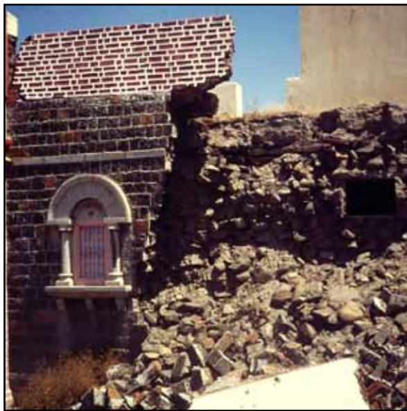
Figure 2.23 Delamination was a common damage pattern observed in the 1993 Maharashtra, India, earthquake (photos: S. Brzev)
