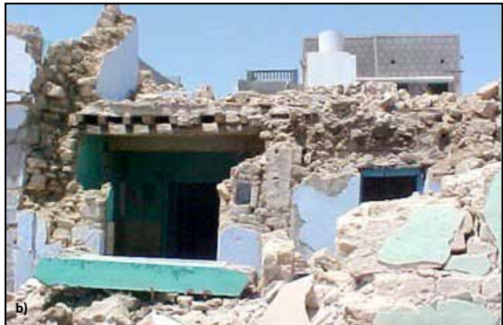
Figure 2.14 Roof deficiencies in the area affected by the 2001 Bhuj, India, earthquake: a) discontinuous rafters over interior walls, and b) inadequate wall-to-floor connections caused the severe building damage (photos: C.V.R. Murty)
