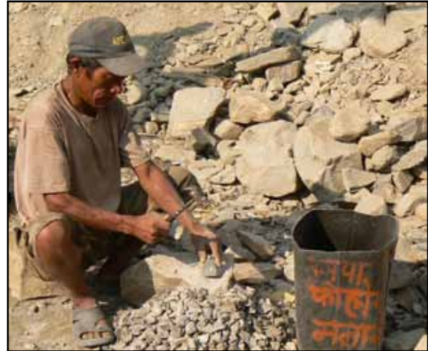
Figure 3.44 Stones can be cut to produce aggregates for concrete construction—an example from Nepal (photo: Smart Shelter Foundation)
