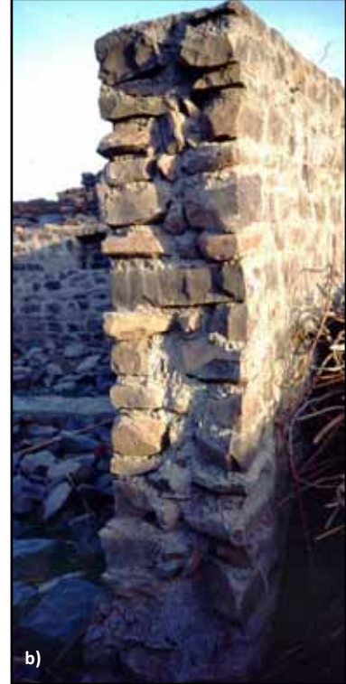
Figure 3.27 Stone masonry in cement mortar with a wall thickness limited to 450 mm (note through-stones) (photos: S. Brzev)
