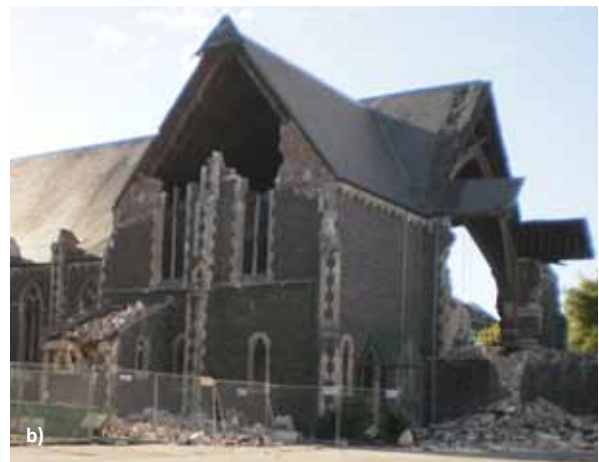
Figure 2.32 Collapse of stone masonry gable walls in New Zealand earthquakes: a) a partial collapse in the 2010 Darfield earthquake, and b) total collapse of the same building in the 2011 Christchurch earthquake (photos: J. Bothara)
