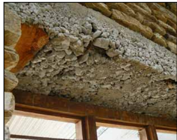
Figure 3.20 Poor concrete construction quality in an RC lintel band (photo: Smart Shelter Foundation)
