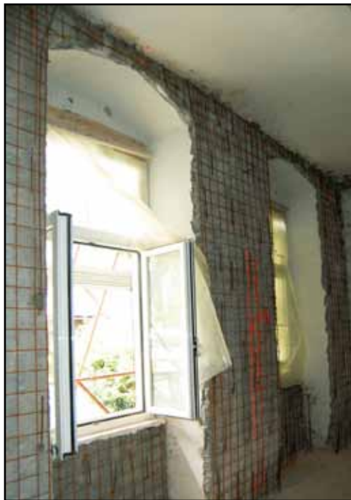
Figure 4.24 Jacketing of a stone masonry wall in Slovenia (photo: M. Lutman)
