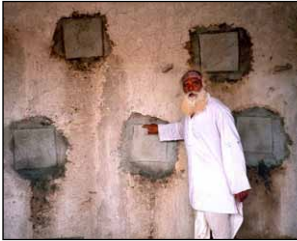
Figure 4.20: Examples of completed through-stone retrofit projects in Maharashtra, India (photos: S. Brzev)
