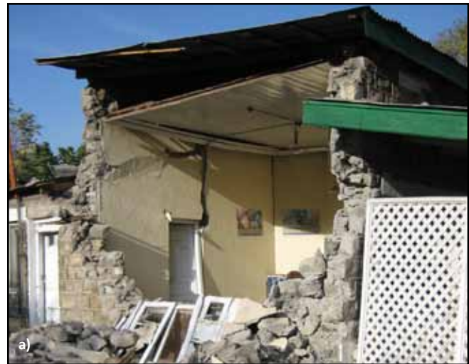
Figure 2.30 Out-of-plane collapse of stone masonry walls in buildings with flexible roofs and inadequate wall-to-roof connections: a) the 2005 Kashmir, Pakistan, earthquake (photo: M. Tomazevic); b) the 2003 Boumerdes, Algeria, earthquake (photo: M. Farsi)
