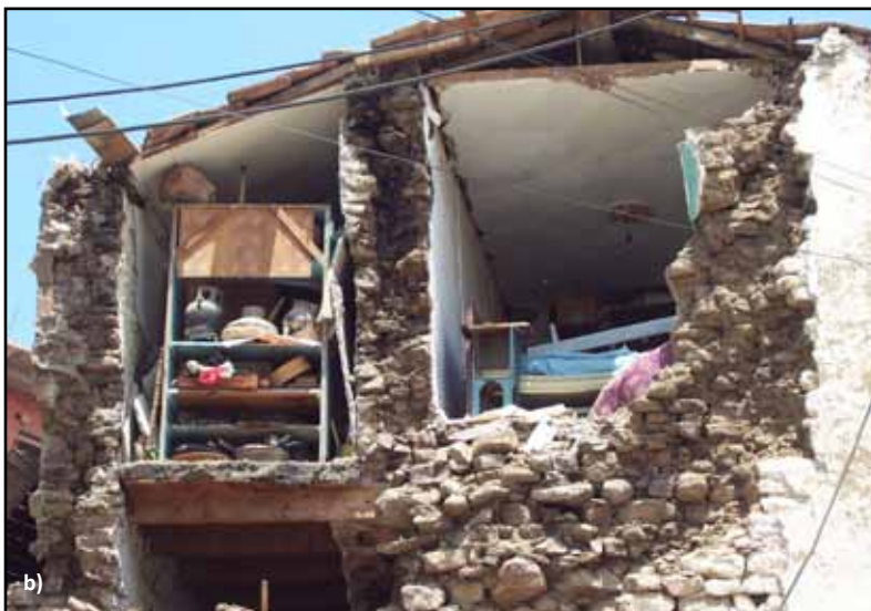
Figure 2.30 Out-of-plane collapse of stone masonry walls in buildings with flexible roofs and inadequate wall-to-roof connections: a) the 2005 Kashmir, Pakistan, earthquake (photo: M. Tomazevic); b) the 2003 Boumerdes, Algeria, earthquake (photo: M. Farsi)
