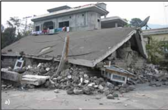
Figure 2.18 Collapse of roof structures due to the loss of gravity load-bearing capacity of stone walls in the 2005 Kashmir, Pakistan, earthquake: a) reinforced concrete roof, and b) timber and steel roof (photos: M. Tomazevic)
