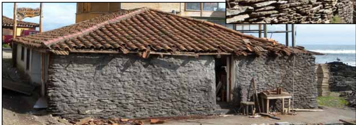
Figure 1.15 A stone masonry house built using slate stones in Duao, Chile (photos: S. Brzev)
