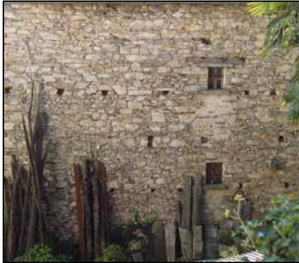
Figure 1.26 Uncoursed semi-dressed stone masonry wall in Southern Switzerland (photo: T. Schacher)
