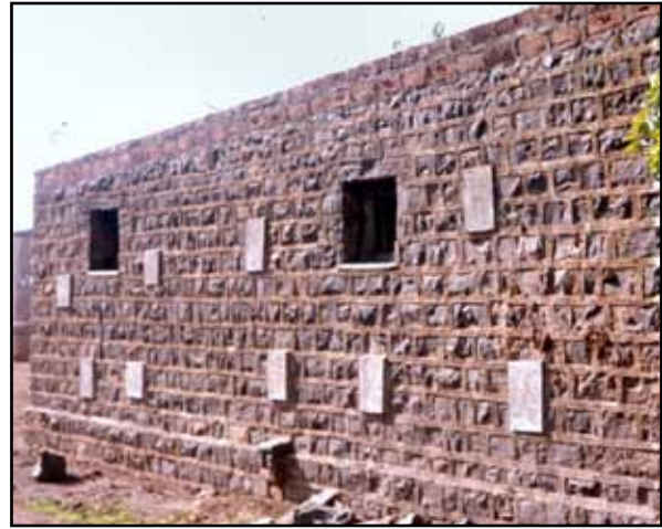
Figure 4.20: Examples of completed through-stone retrofit projects in Maharashtra, India (photos: S. Brzev)
