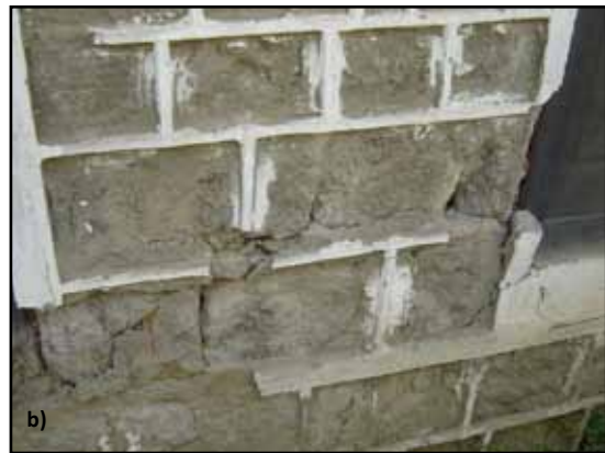
Figure 2.34 Shear failure in stone masonry walls: a) shear cracks initiated at the corners of openings in the 2005 Kashmir, Pakistan, earthquake (Photo: Bothara and Hiçyılmaz, 2008), and b) shear cracking in a stone masonry pier damaged by the same earthquake (photo: Builders Without Borders)
