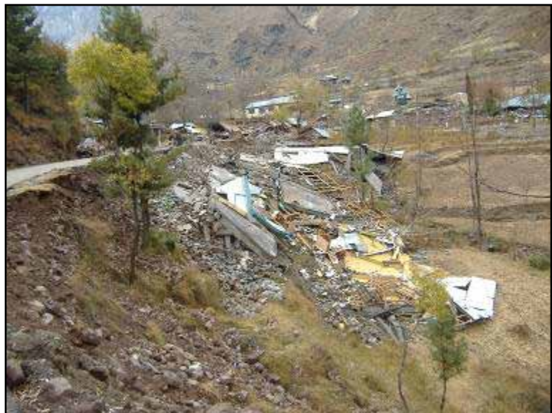
Figure 3.1 A collapsed building on a steep slope after the 2005 Kashmir earthquake, Pakistan (source: Bothara and Hıçyılmaz 2008)
