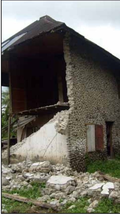
Figure 2.29 (left and above) Out-of-plane collapse of stone masonry walls in the 2009 Padang, Indonesia, earthquake (source: Bothara et al. 2010)
