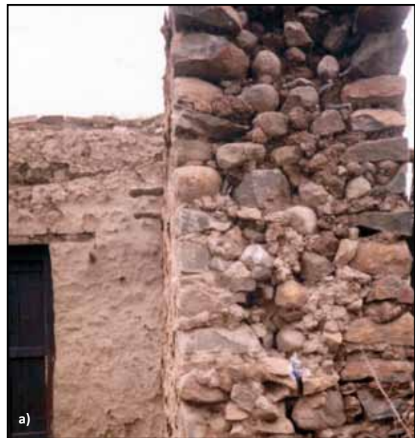
Figure 1.22 Typical uncoursed random rubble stone walls: a) an uncoursed random rubble stone wall in Maharashtra, India, showing exterior wythes and stone rubble in mud mortar in between (photo: S. Brzev) and b) plan view of a stone wall under construction in Nepal (note stone rubble between the wall wythes) (photo: Smart Shelter Foundation)
