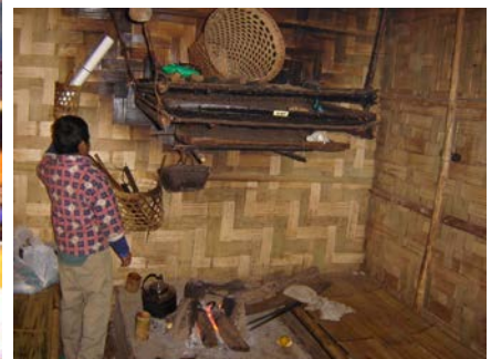
Loft above the hearth - is used to dry the firewood and to store utensils etc.
