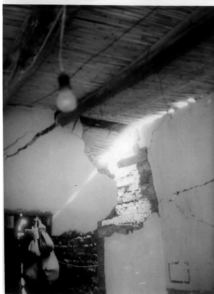
Figure 7: Damage in the 1977 Caucete Earthquake Figure 8: Damage in the 1977 Caucete Earthquake Figure 9: Damage in the 1977 Caucete Earthquake
