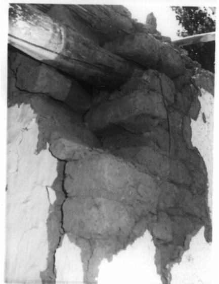
Figure 7: Damage in the 1977 Caucete Earthquake Figure 8: Damage in the 1977 Caucete Earthquake Figure 9: Damage in the 1977 Caucete Earthquake
