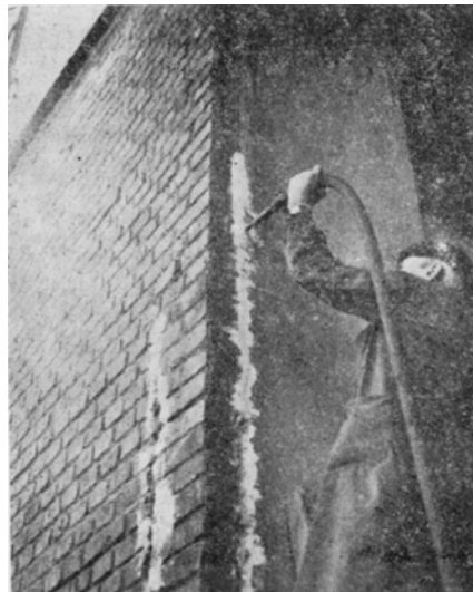
Figure 25: Wall repair by injecting cement paste
