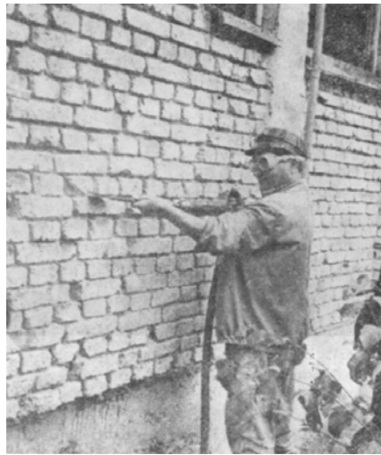
Figure 28: Torcrete method - step 1: cleaning of the wall surface with compressed air
