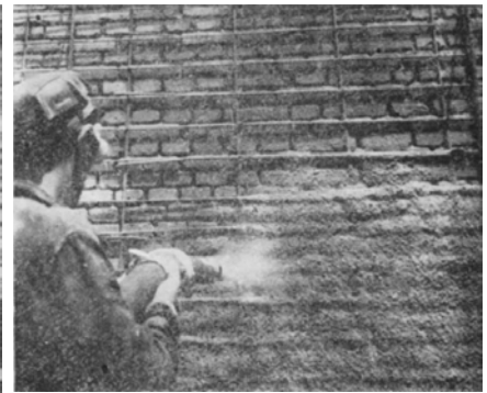
Figure 29: "Torcrete" retrofit : application of torcrete overlay on the steel net attached to the wall
