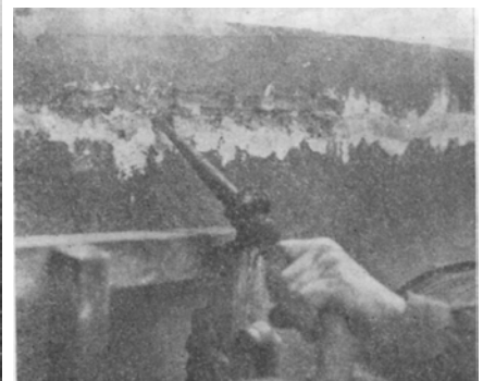
Figure 26: Wall repair by injecting cement paste with compressed air
