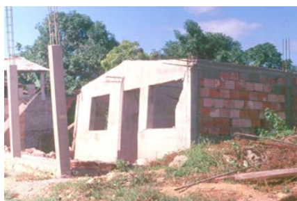
Figure 6: A Photograph Illustrating Typical Damage (1997 Caríaco earthquake)
