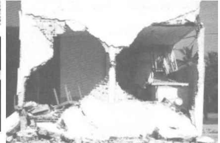
Figure 6C: Typical earthquake damage: collapse of a confined wall (1985 Lolleo earthquake)
