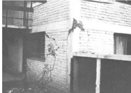
Figure 6B: Typical earthquake damage: cracking of concrete posts and masonry walls (1985 Lolleo earthquake)
