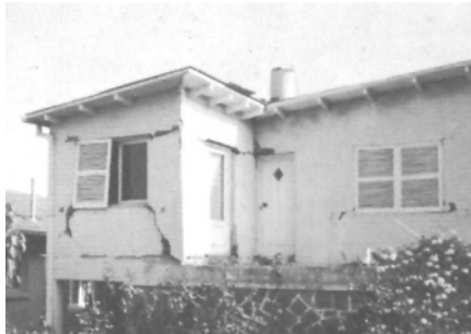
Figure 6D: Typical earthquake damage: cracking of masonry walls (1985 Lolleo earthquake)
