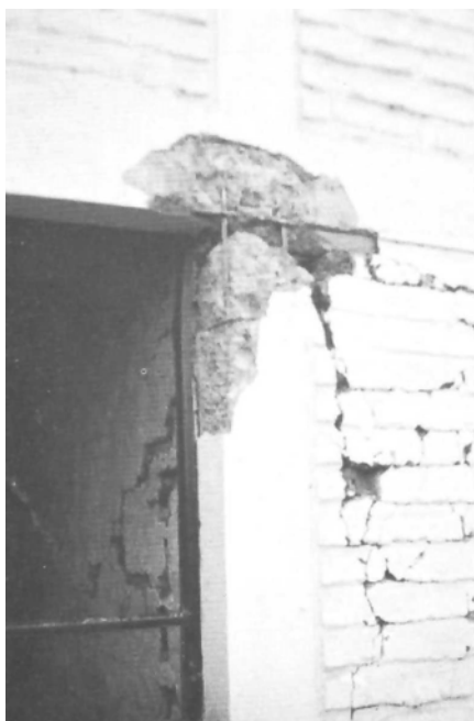
Figure 6: Typical earthquake damage: cracking of
