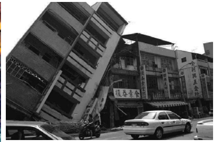
Figure 6F: Collapse of a Concrete Frame Building in the 1999 Chi Chi Earthquake (Source: EERI 2001)
