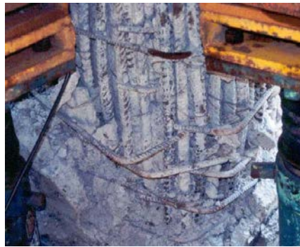
Figure 6E: Earthquake Damage - Opening of 90 degree column hooks in the 1999 Chi Chi earthquake (Source: EERI 2001)
