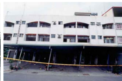
Figure 6C: Earthquake Damage - Partial Collapse of a Three-story building in the 1999 Chi Chi Earthquake (Source: EERI 2001)
