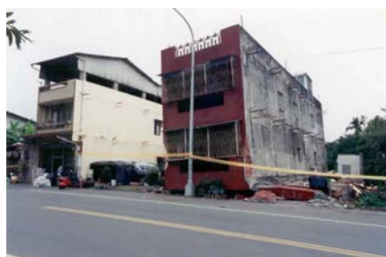
Figure 6B: Earthquake damage-Collapsed Three-story building in the 1999 Chi Chi earthquake (Source: EERI 2001)
