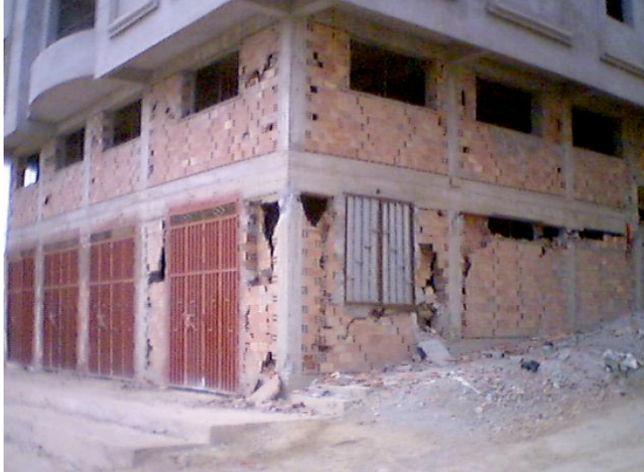
Fig. 6: Damaged column and soft storey damage (grade 4 vulnerability C)
