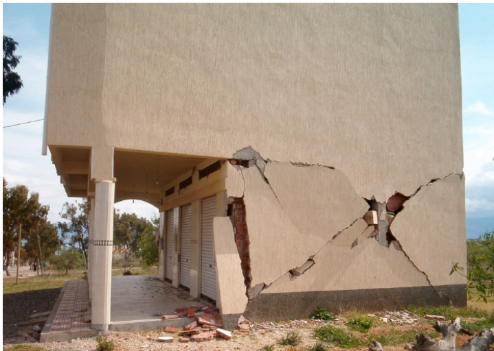
Fig. 4: Soft storey damage to this RC building in Al Hoceima region. (grade 3 vulnerability C)
