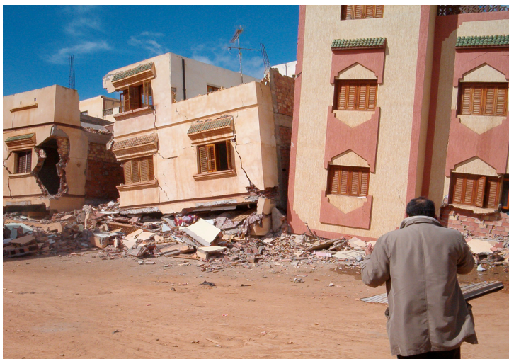
Fig. 5: On the right: building with ground floor collapse (grade 5 vulnerability C) On the left: both ground and first floors failed in this building (grade 5 vulnerability C)
