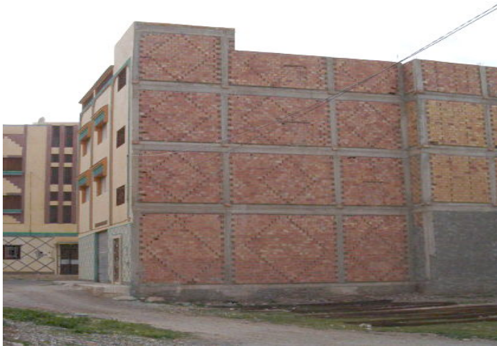
Fig. 7: Shear damage to the hollow brick wall with RC frame (grade 2 vulnerability C)
