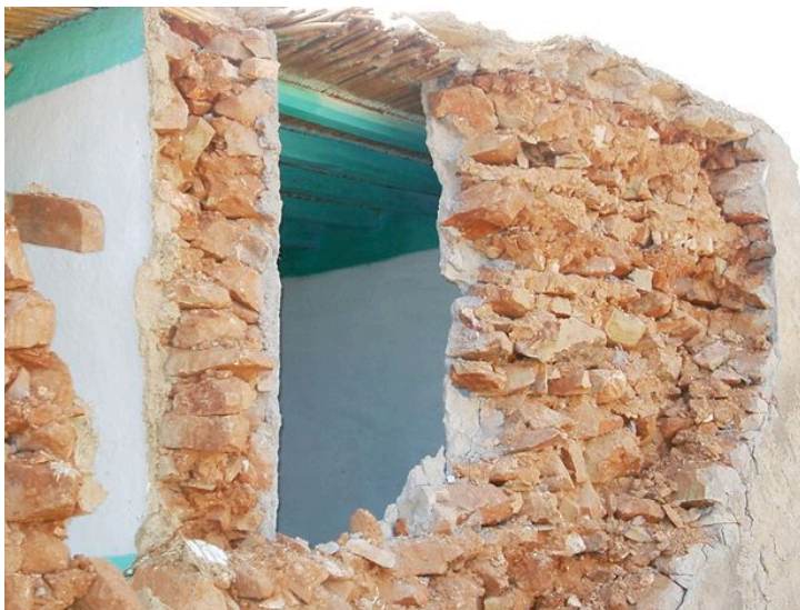
Fig. 8: Advanced corner failure of traditional masonry. Rural area in Al Hoceima region (grade 4 vulnerability A)
