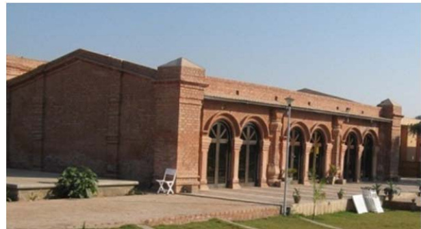
Figure 4. Khazana – a cultural center/library in Khairpur. Arcaded brick construction.
