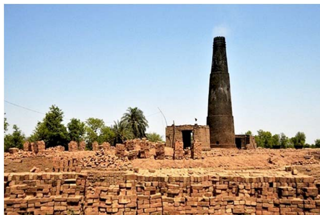
Figure 1. Typical brick kiln to produce fired bricks in Punjab.
