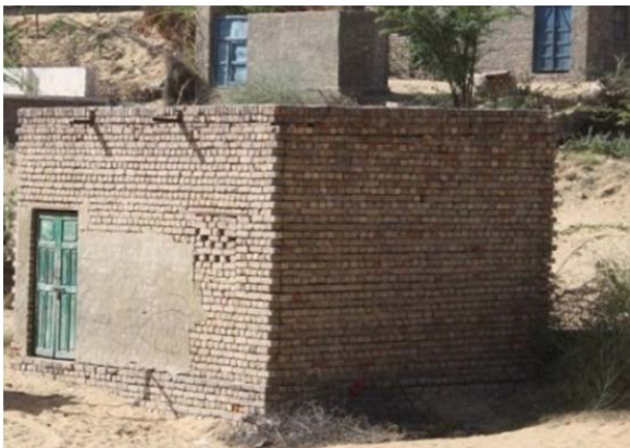
Figure 3. Rural brick houses – Mithi, Thar.
