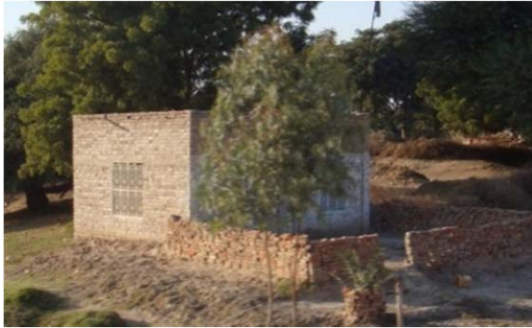
Figure 5. A small, one-room roadside brick mosque.
