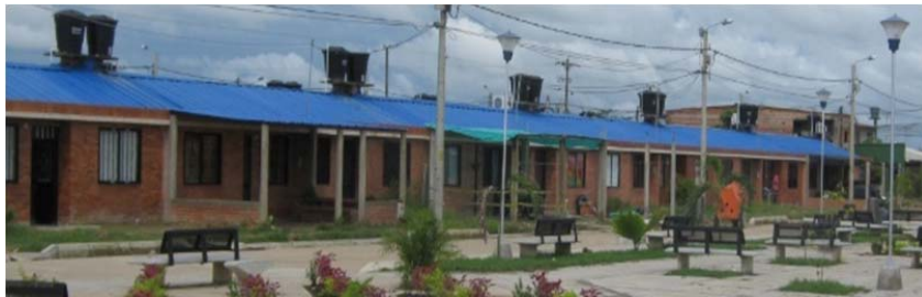
Figure 1. Typical one-story house (August 2011) [1].
