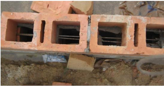
Figure 9. Horizontal reinforcement placed in between the horizontal bed joints. (2 bars of 4mm diameter) (August 2011) [1].
