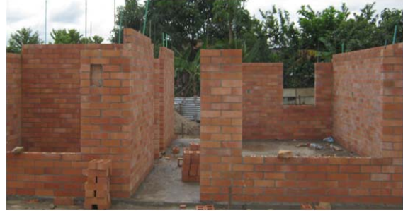
Figure 8. Reinforced masonry walls' assembly after the mat foundation. (August 2011) [1].
