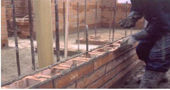
Figure 7. Location of the reinforcement and application of the mortar [2].
