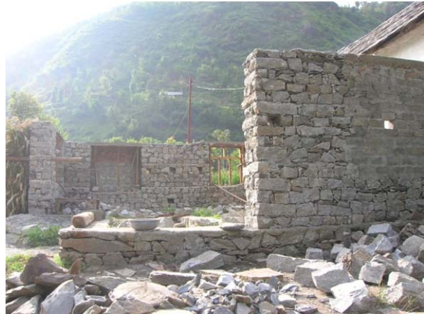
Figure 9. Plinth level of a house under construction.
