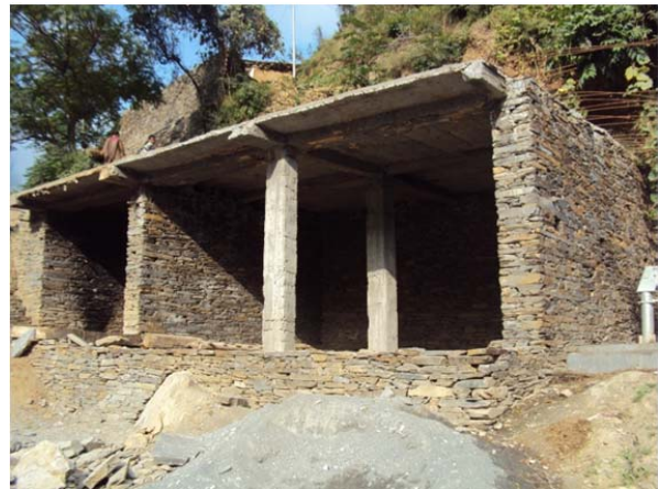
Figure 7. A dry stone structure with RC flat slab under construction. RC columns are additionally used to support the longer span.
