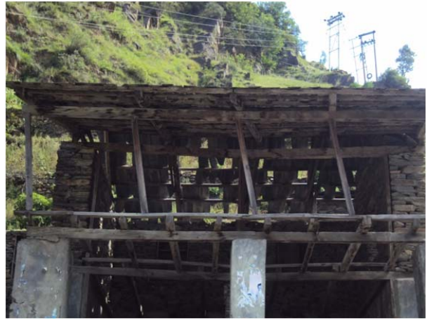
Figure 13. Secondary wooden members resting on the main wooden beam in order to construct the first floor.
