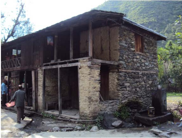
Figure 12. A house showing its exposed exterior and plastered interior.
