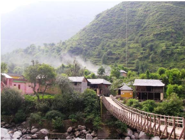
Figure 14. View of village Rakh, in Chamba district with a variety of dry stone masonry houses; gable-end roof, hipped roof and roof-changing-angle over verandah can be seen.
