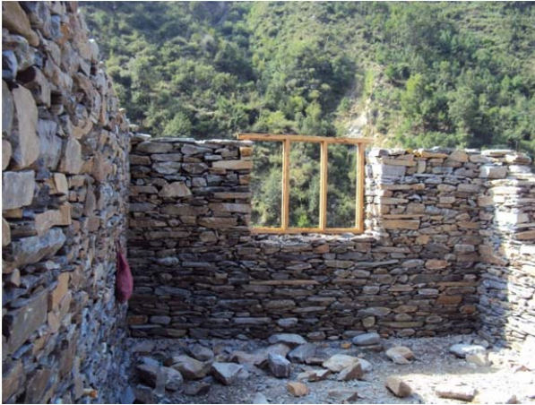
Figure 4. Large opening in wall for light and ventilation purpose.
