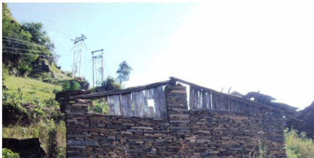
Figure 16. Gable-end roof where wooden planks have been used as gable infill.
