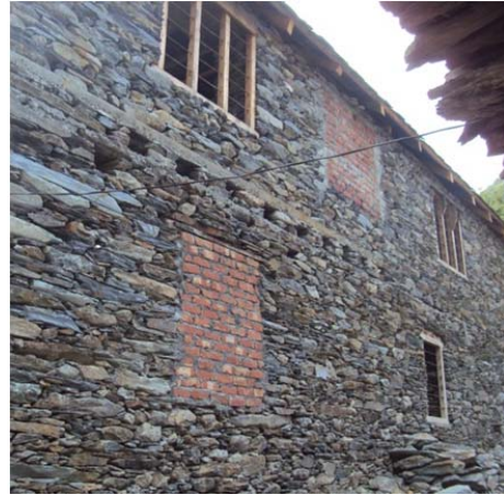
Figure 5. Use of bricks to accommodate cupboards at the inside of the wall.
