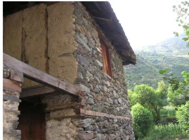
Figure 11. Wooden beam at lintel/floor level.
