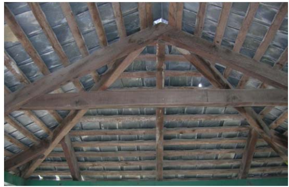
Figure 15. A-type frame of a hipped roof.
