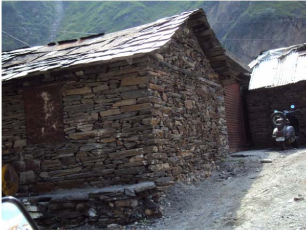
Figure 8. Raised plinth of a house can be seen in the front.
