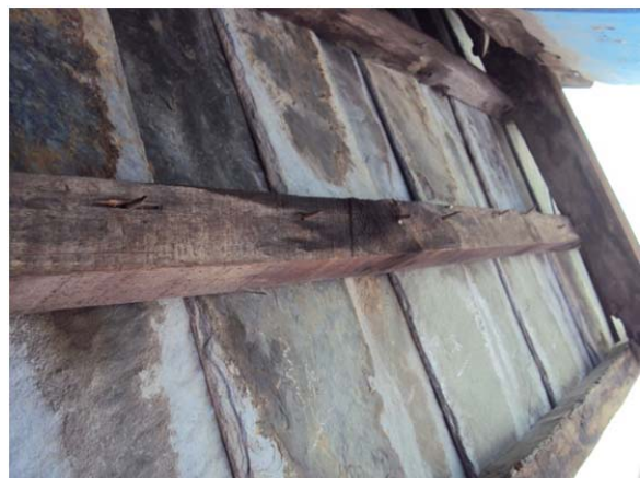
Figure 17. Slates nailed to the roof purlin.
