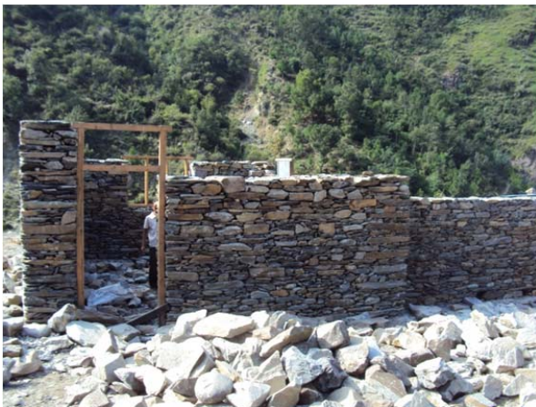
Figure 10. A house under construction illustrating the width of the walls as well as the varying sized stones.
