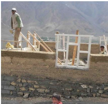
Figure 19. Walls with already placed window frames.
