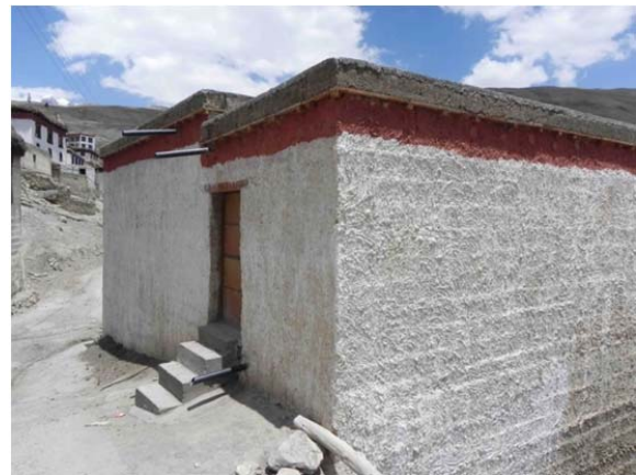
Figure 20. Patterns made to the outer walls with mud slurry for finishing.
