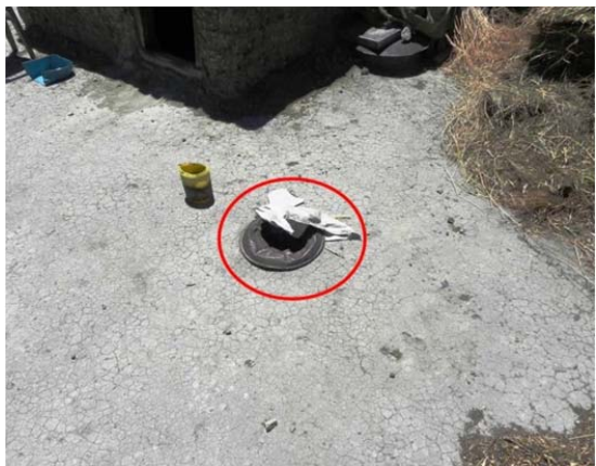
Figure 7. Sky-light as seen from terrace.
