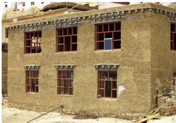
Figure 10. Precast RC lintels in a new construction.
