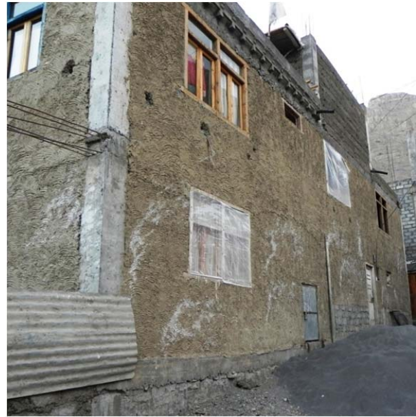
Figure 12. RC framed structure with mud walls infill and mud roof.
