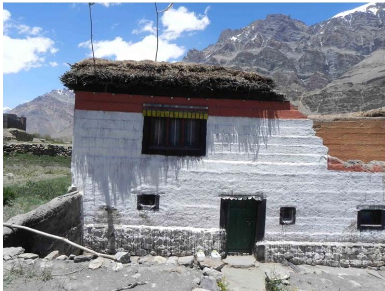
Figure 13. Lower portion of the wall made up of field stones. The front door is arranged at ground floor level without any plinth.
