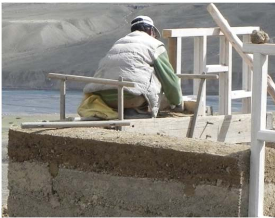
Figure 17. Wooden formwork to lay courses of mud.
