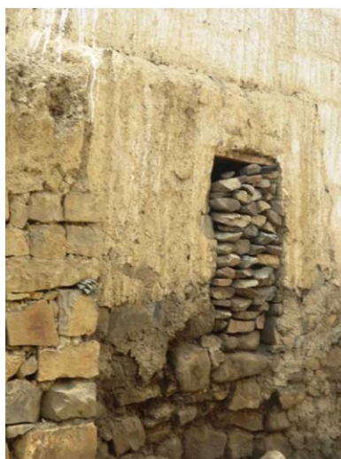
Figure 16. Septic tank's opening closed with dry stone packing.
