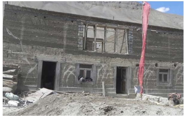
Figure 18. Marks can be seen on the wall of the upper floor where windows have to be cut. Lintel beams have already been provided during the wall construction process.
