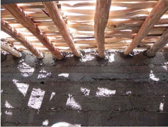
Figure 21. Branches are densely laid over poplar tree logs (beams).
