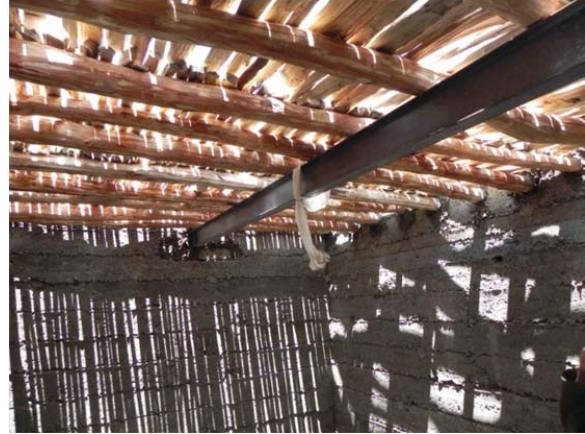
Figure 22. A steel I-section girder is used to support the beams.
