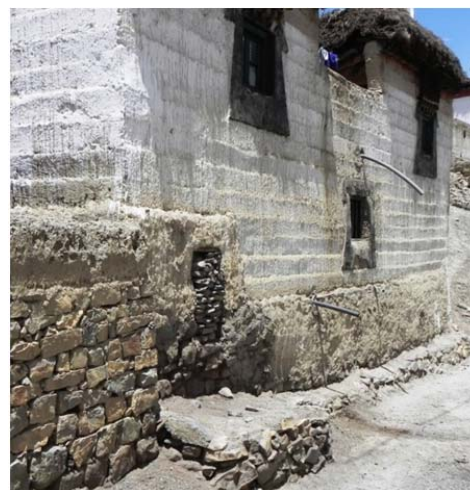
Figure 15. Over-ground septic tank's opening can be seen at ground floor level.
