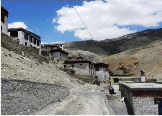
Figure 5. Houses located on slopes.
