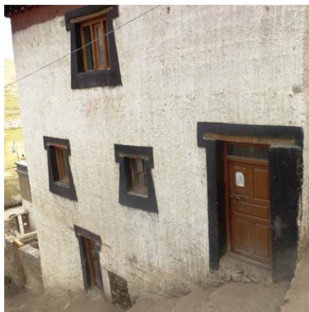
Figure 9. Doors at different levels.
