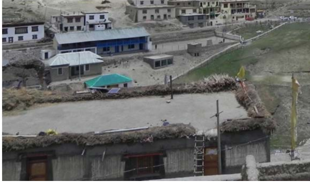
Figure 23. Parapet over a Spitian house terrace.
