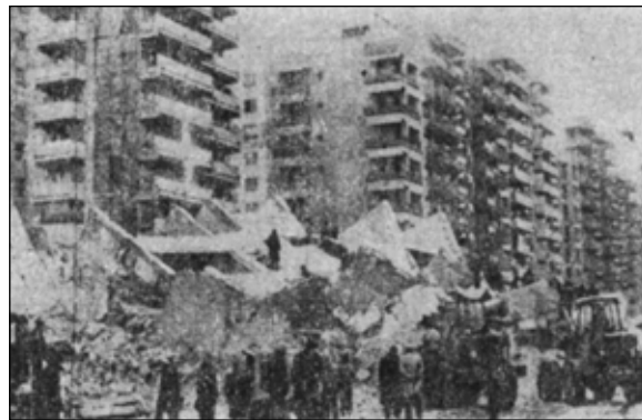
Figure 5: Building collapse in 1977 Vrancea earthquake (WHE Report 78, Romania)
