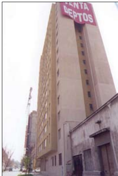
Figure 1: Typical building in Chile (WHE Report 4)
