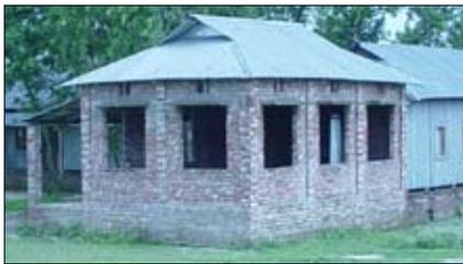
Figure 1: One-story brickwork construction in Bangladesh (WHE Report 91)
