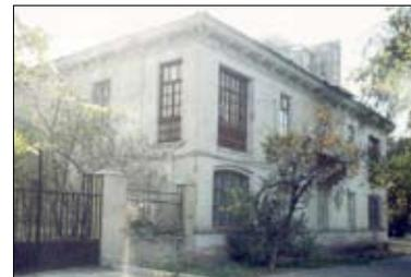
Figure 2: Two-story brick masonry building with wooden floors (WHE Report 41, Kyrgyzstan)
