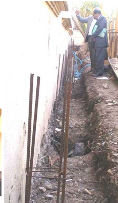
Figure 6C: Seismic Strengthening Techniques: Construction of RC Ties
