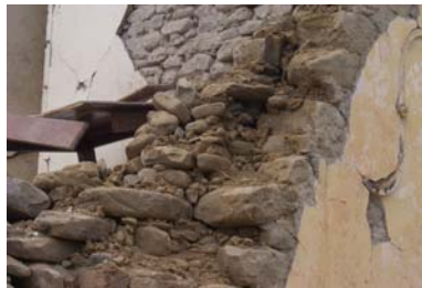
Figure 5E: Collapse of a roof and a side wall na multi-storey stone masonry building in Algiers city in the May 21, 2003 earthquake
