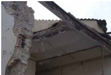
Figure 5D: Damage to a stone masonry building in Algiers in the May 21, 2003 earthquake
