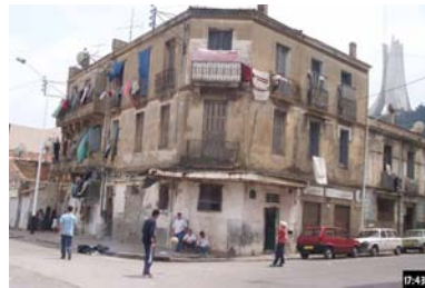
Figure 1B: A typical old stone masonry building in Algiers city
