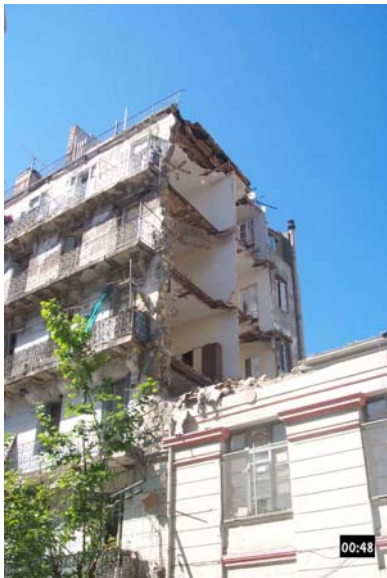
Figure 5A: Typical Earthquake Damage: Partial Roof Collapse (1999 Ain-Temouchent Earthquake)
