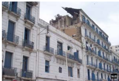
Figure 5E: Collapse of a roof and a side wall na multi-storey stone masonry building in Algiers city in the May 21, 2003 earthquake
