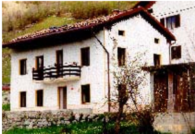
Figure 1A: Typical Building
