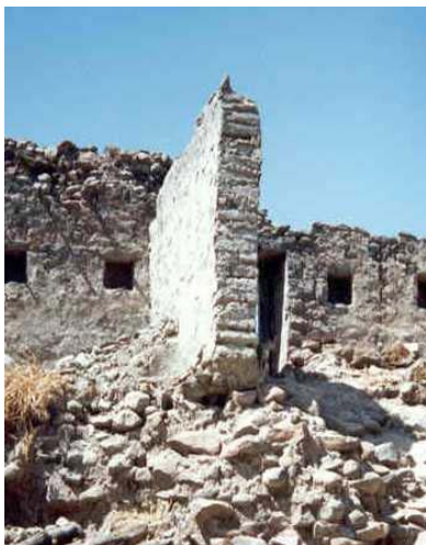
Figure 5: Key Seismic Deficiency - Extremely Thick Stone Walls
