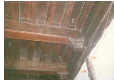
Figure 4B: Critical Structural Details - Good Quality Timber Roof Structure
