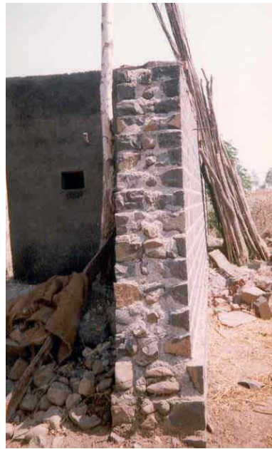
Figure 5A: Seismic Resilient Feature - Well Constructed Stone Wall
