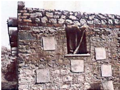
Figure 7F: Seismic Strengthening - Installation of Through Stones (Source: GOM 1998)
