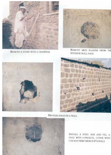
Figure 7G: Seismic Strengthening - A Field Application of Through Stones (Source: GOM 1998)
