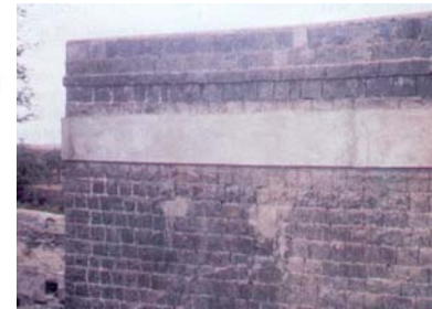
Figure 7E: Seismic Strengthening - Installation of Through Stones (Source: GOM 1998)
