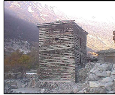
Figure 5 (b): A historical three story building, with single room at each floor; well standing the past seismic events.
