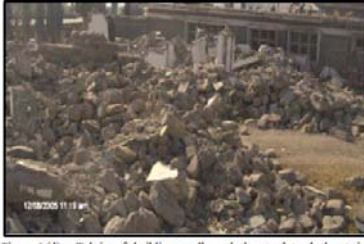
Figure 6 (d): Debris of buildings collapsed due to lateral thrust in addition to seismic forces. Note a building in the background with rigid diaphragm is still standing, Pakistan earthquake of October 08, 2005.
