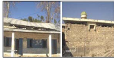
Figure 6 (f): Slippage of top course of masonry; Pakistan earthquake of October 08, 2005.
