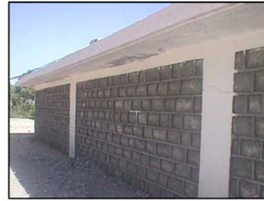
Figure 1 (g): A view of stone masonry house constructed with dressed stones in cement sand mortar having R.C.C. roof.
