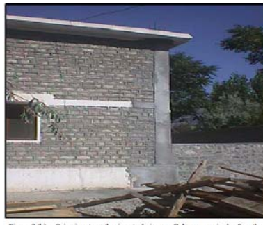
Figure 7 (b): Seismic strengthening techniques; Column repaired after the earthquake.
