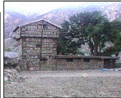
Figure 7 (c): Seismic strengthening techniques; Horizontal and Vertical wooden bands introduced after the earthquake.
