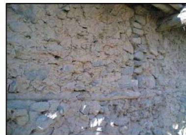
Figure 1 (c): A view of typical stone masonry wall constructed in mud mortar.
