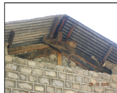
Figure 6 (c): Gable wall failure: Pakistan earthquake of October 08, 2005.
