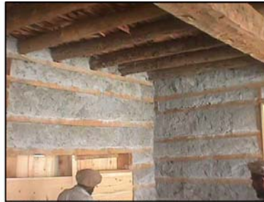
Figure 5 (d): Inner close view of building in fig 5 c.
