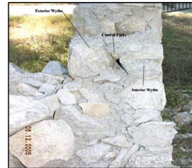
Figure 4 (b): Typical wall section; photo of a damage wall from October 08, 2005 earthquake 2005; two wythes & central portion of wall are clearly visible.
