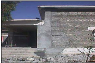
Figure 7 (a): Seismic strengthening technique; Column repaired after the earthquake.
