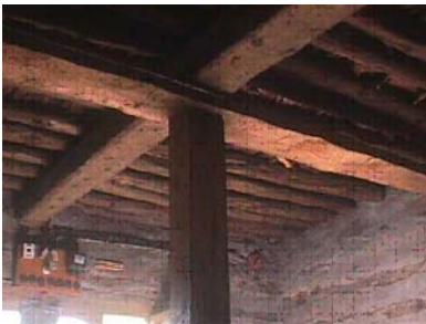
Figure 7: A wooden column in the center of a room, in addition to the main stone masonry walls, is provided to support roof gravity load
