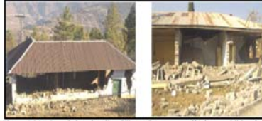
Figure 6 (e): Out of plane bending failure of masonry walls due to additional thrust from roof trusses; Pakistan earthquake of October 08, 2005.
