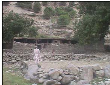
Figure 6 (b): Out-of-plane failure of stone masonry in dry, Pakistan earthquake of October 08, 2005
