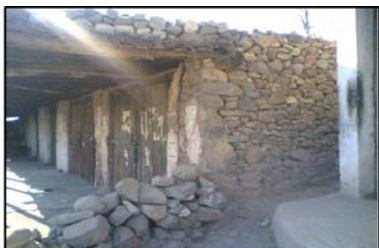
Figure 1 (a): A view of typical stone masonry house constructed in dry (without any mortar) with earthen roof.
