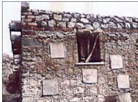
Figure 8: The application of through-stones as practiced in India (WHE Report 18)
