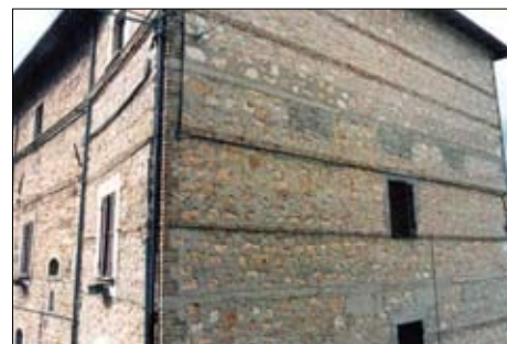
Figure 10: Seismic-strengthening techniques in Italy: installation of new steel wall ties (WHE Report 28)
