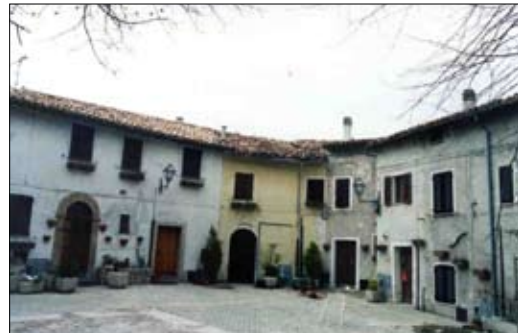
Figure 2: Single-family stone masonry house in Italy (WHE Report 28)
