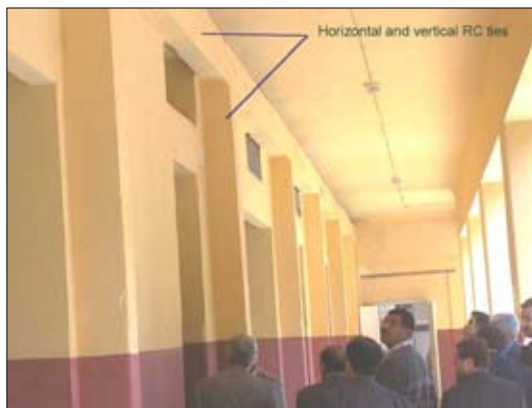
Figure 11: An example of a strengthened building with vertical and horizontal reinforced concrete ties at the first floor level as practiced in Algeria (WHE Report 75)
