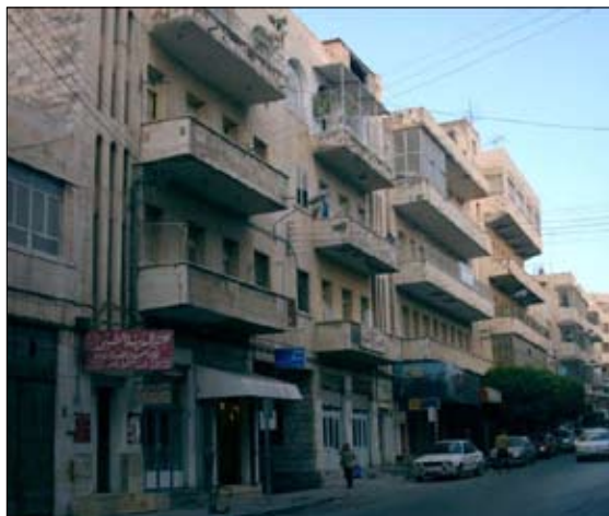
Figure 3: Unreinforced concrete and stone masonry building in the Palestinian Territories (WHE Report 49)
