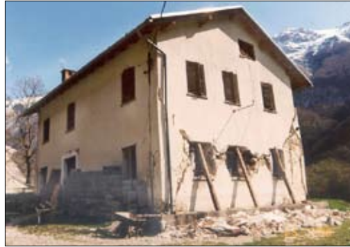
Figure 7: Typical damage during the 1998 Bovec earthquake in Slovenia (WHE Report 58)
