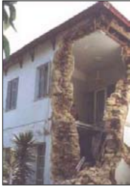
Figure 6: Typical collapse of a corner (WHE Report 16, Greece)
