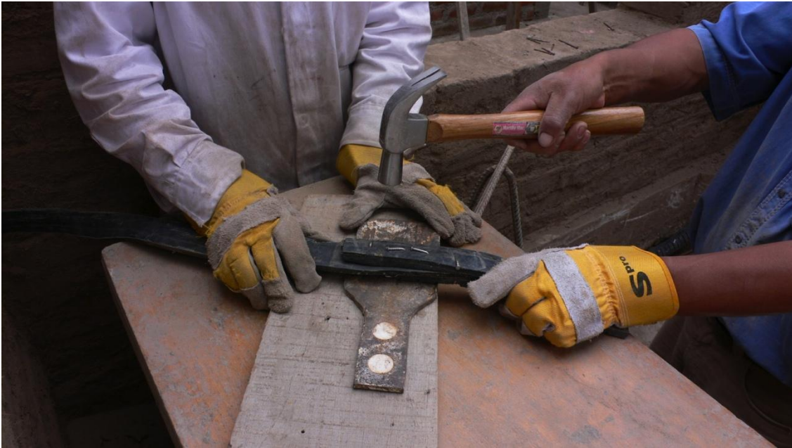
Figure 4.5 A firm support and a steel plate assist the nailing and nail bending process.
