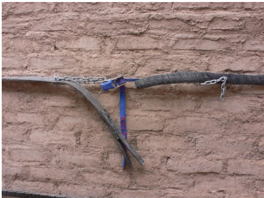
Figure 4.19 Strap is tensioned with the half pre-nailed joint hanging down. The right-hand end of the strap requires shortening.
