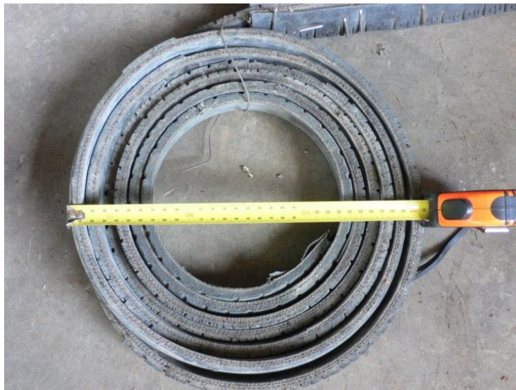
Figure 1.2 A tire strap approximately 6 m long ready to be applied to a house.
