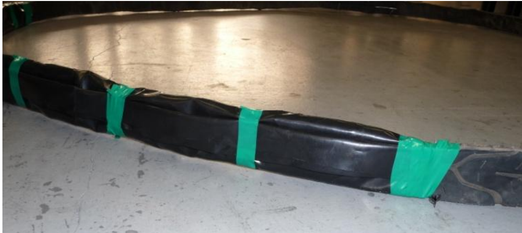
Figure 4.7 A strap with a length of PVC sheet to provide water protection to the strap below ground level and up to the height where the strap is protected by mud mortar and painted surfaces.
