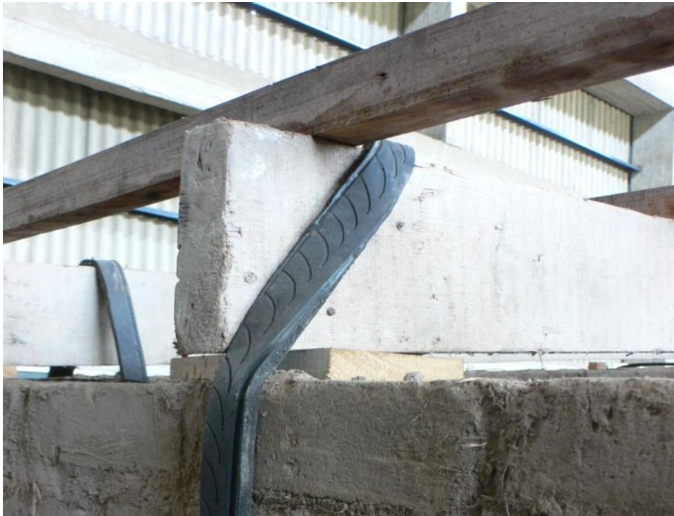
Figure 4.10 A strap wrapping over a rafter. In this trial house the straps were not placed in wall rebates and the rafters were not notched.
