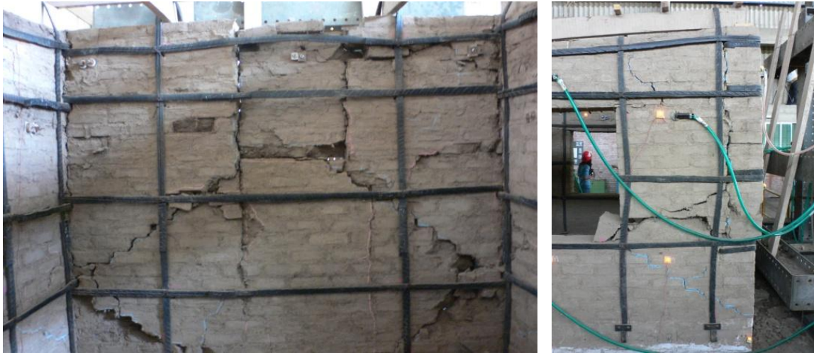
Figure A.6 Damage to the rear wall after the Phase 3 (maximum shaking) (left) and the most heavily damaged pier.
