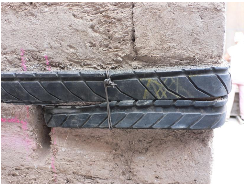
Figure 4.22 Two straps around an exterior corner. The upper edge of the top strap is aligned with the horizontal mortar joint. The horizontal joint between the two straps is therefore approximately mid-height of an adobe block. Note that the hole for the lower strap is deeper vertically than necessary.
