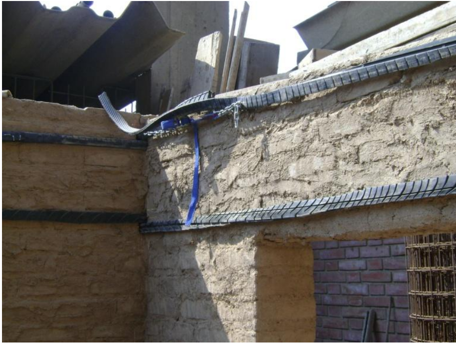
Figure 4.18 The upper strap is taut but requires shortening using a hacksaw before nailing the joint.
