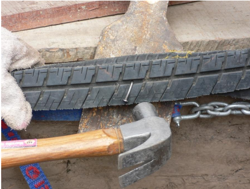
Figure 4.21 After using a wooden backing block to drive a nail half-way through, a steel plate helps bend the nail down on the back of a strap.
