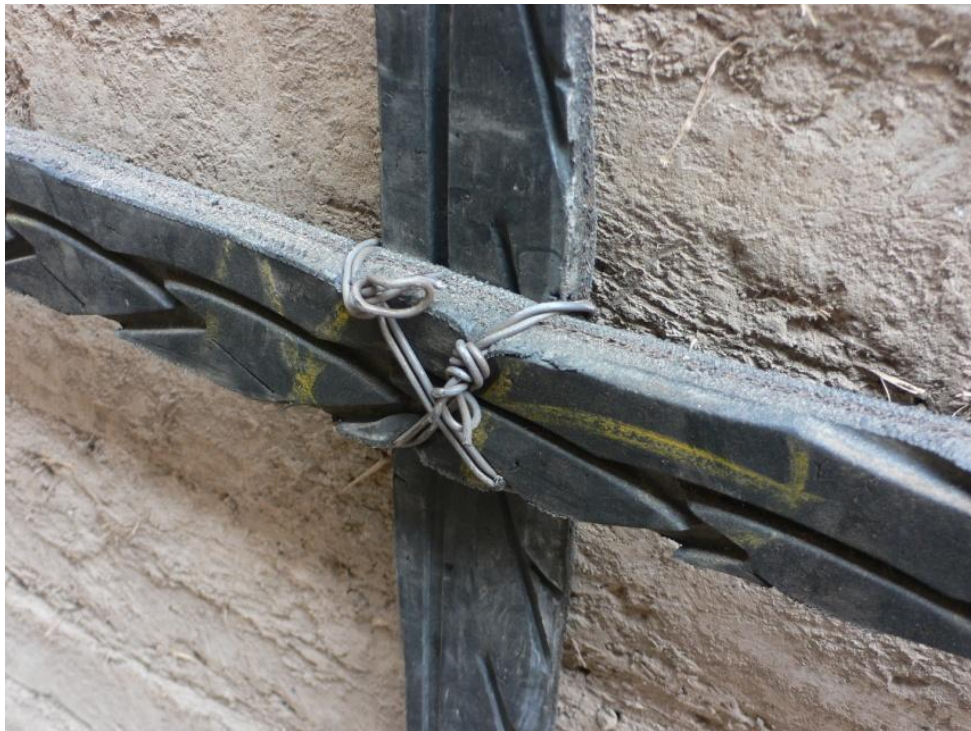
Figure 4.30 A strap junction tied together and through the wall tightly by a pair of tie wires.
