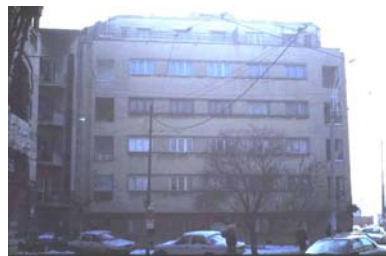
Figure 1B: Typical Building
