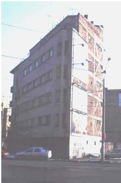
Figure 1A: Typical Building
