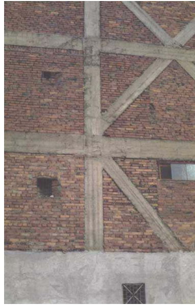
Figure 4B: Critical Structural Details - Frame with Diagonal Braces and Masonry Infill
