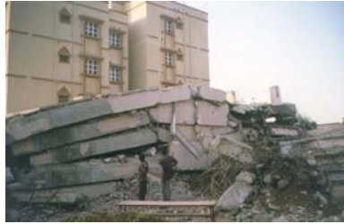
Figure 6E: Damage to Ground Floor Columns Due to Inadequate Lateral Confinement of Reinforcement Bars
