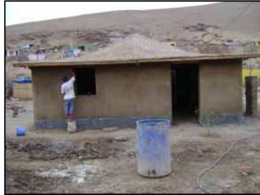
Figure 3.9 Mud plaster on an adobe house
