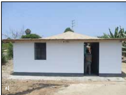
Figure 4.14 Reinforced adobe houses in Chincha, Peru built after the 2007 Pisco earthquake: a) A model house from PUCP-CARE's booklet, and b) Reinforced adobe house built by CARE
