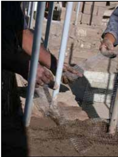
Figure 4.5 Construction of an adobe building with internal PVC tubes and plastic mesh
