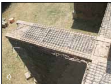
Figure 4.11 Construction details for the geomesh reinforcing scheme: a) Geomesh anchored to the foundation, b) Geomesh attached to adobe walls, c) Geomesh attached to the ring beam, and d) Geomesh covered with mud plaster
