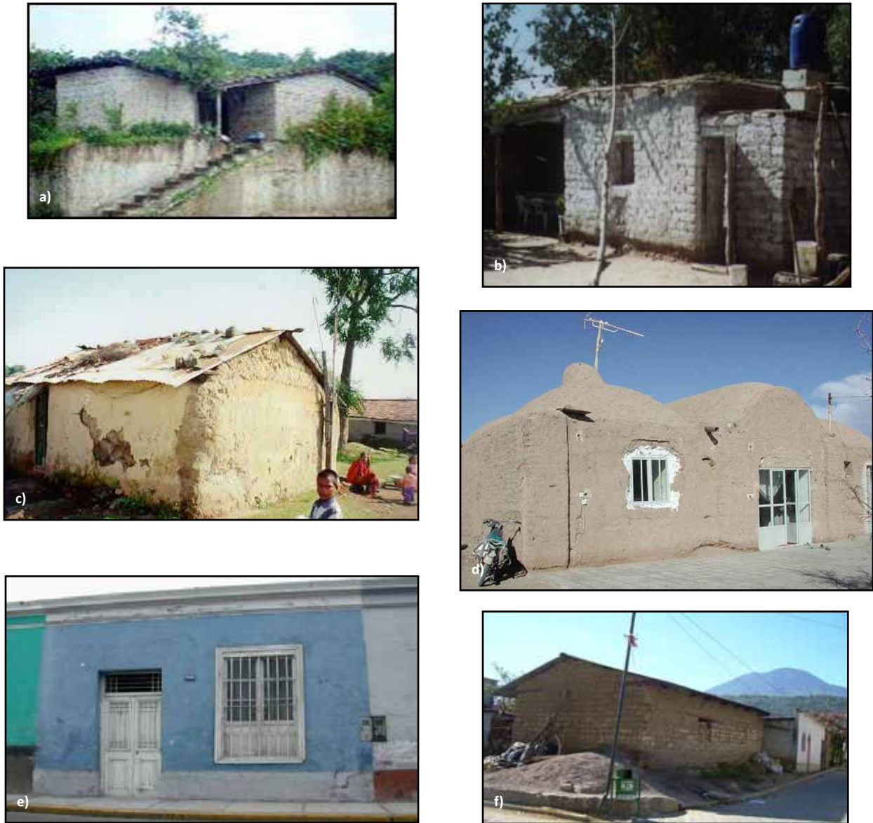
Figure 1.3 Typical adobe houses around the world: a) El Salvador (source: Lopez et al. 2002), b) Argentina (source: Rodriguez et al. 2002), c) India (source: Kumar 2002), d) Iran (source: Mehraim and Naeim 2004), e) Peru (source: Loaiza et al. 2002), and f) Guatemala (source: Lang et al. 2007)
