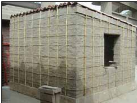
Figure 4.6 An adobe building model with external vertical cane and horizontal rope reinforcement
