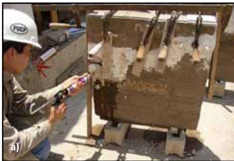
Figure 5.2 Grout injection procedure: a) Crack injection, and b) Repaired wall
