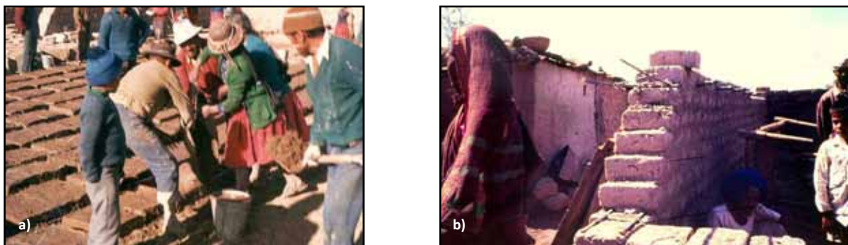
Figure 1.4 Adobe construction performed by local communities: a) Block making in Peru (photo: M. Blondet), and b) Building construction in India (photo: S. Brzev)
