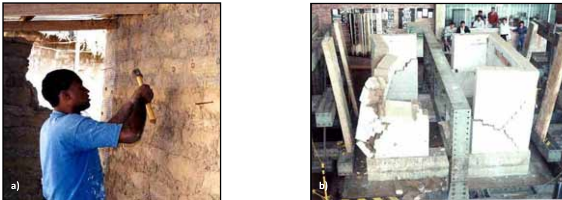
Figure 4.8 Welded wire mesh reinforcement: a) Mesh installation, and b) Shake table testing of U-shaped walls
