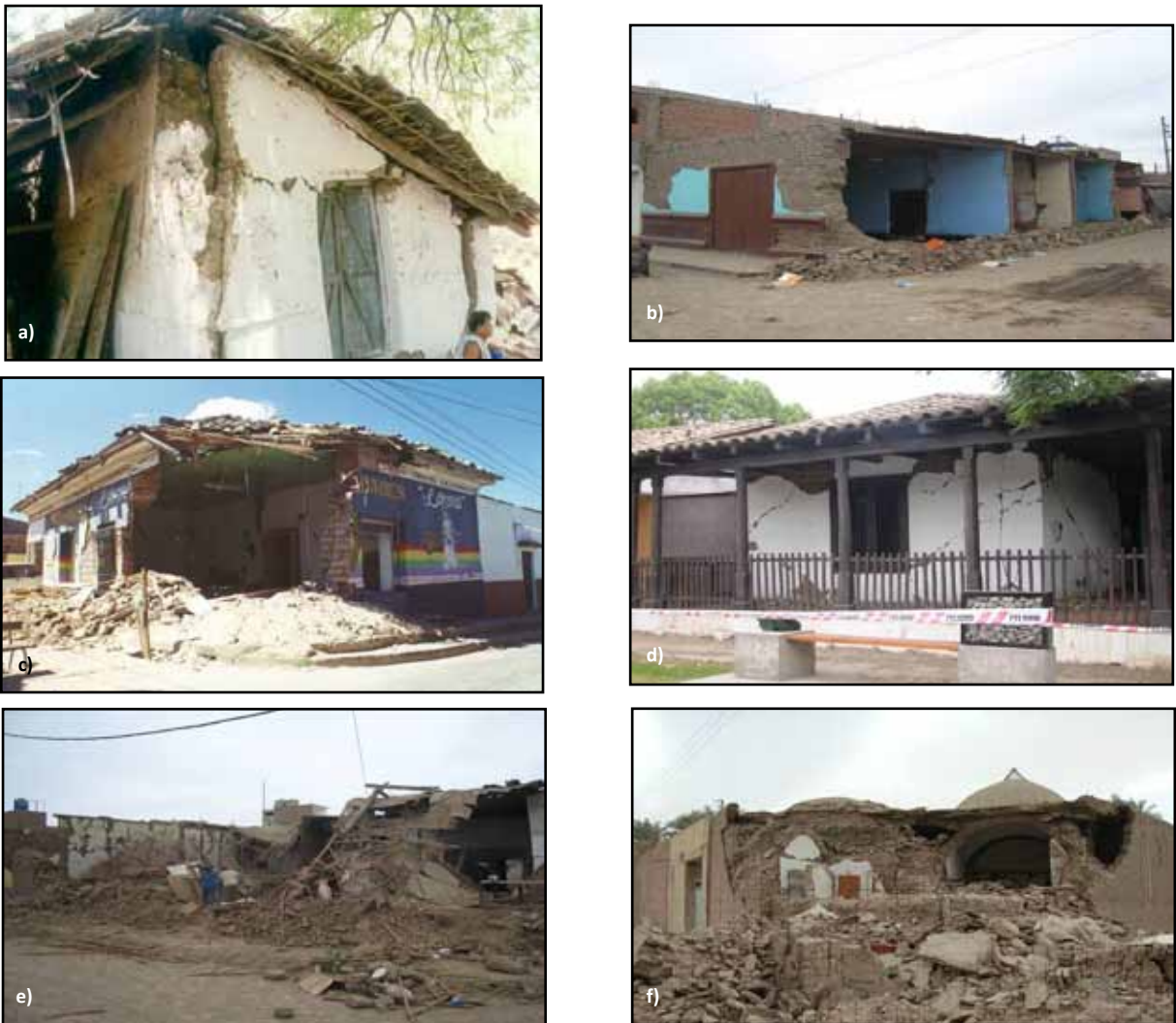
Figure 2.3 Typical patterns of earthquake damage in adobe walls: a) Vertical cracking and separation of adobe walls after the 1997 Jabalpur, India earthquake (source: Kumar 2002), b) Out-of-plane wall collapse after the 2007 Pisco, Peru earthquake (photo: M. Blondet), c) Total collapse of adobe walls after the 2001 El Salvador earthquake (source: Lopez et al. 2002), d) Diagonal cracking of adobe walls after the 2010 El Maule, Chile earthquake (source: Astroza et al. 2010), e) Roof collapse on an adobe building after the 2007 Pisco, Peru earthquake (photo: M. Blondet), and f) Parapet collapse on an adobe building after the 2003 Bam, Iran earthquake (source: Mehraïn and Naeim 2004)
