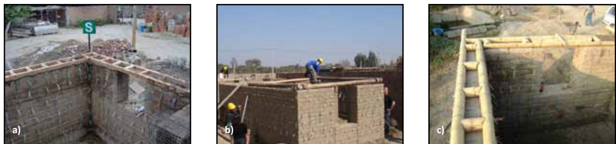
Figure 4.1 Ring beams made of different materials: a) Wood, b) Eucalyptus logs, and c) Bamboo
