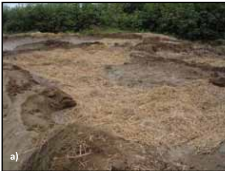
Figure 3.3 Adding straw to the soil: a) Straw to be added, and b) Mixing the straw and soil
