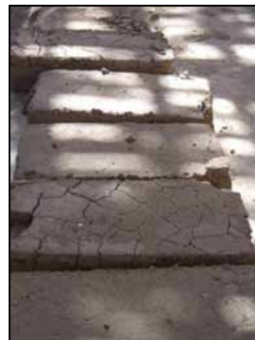
Figure 3.4 Opened “sandwiches” with visible cracking
