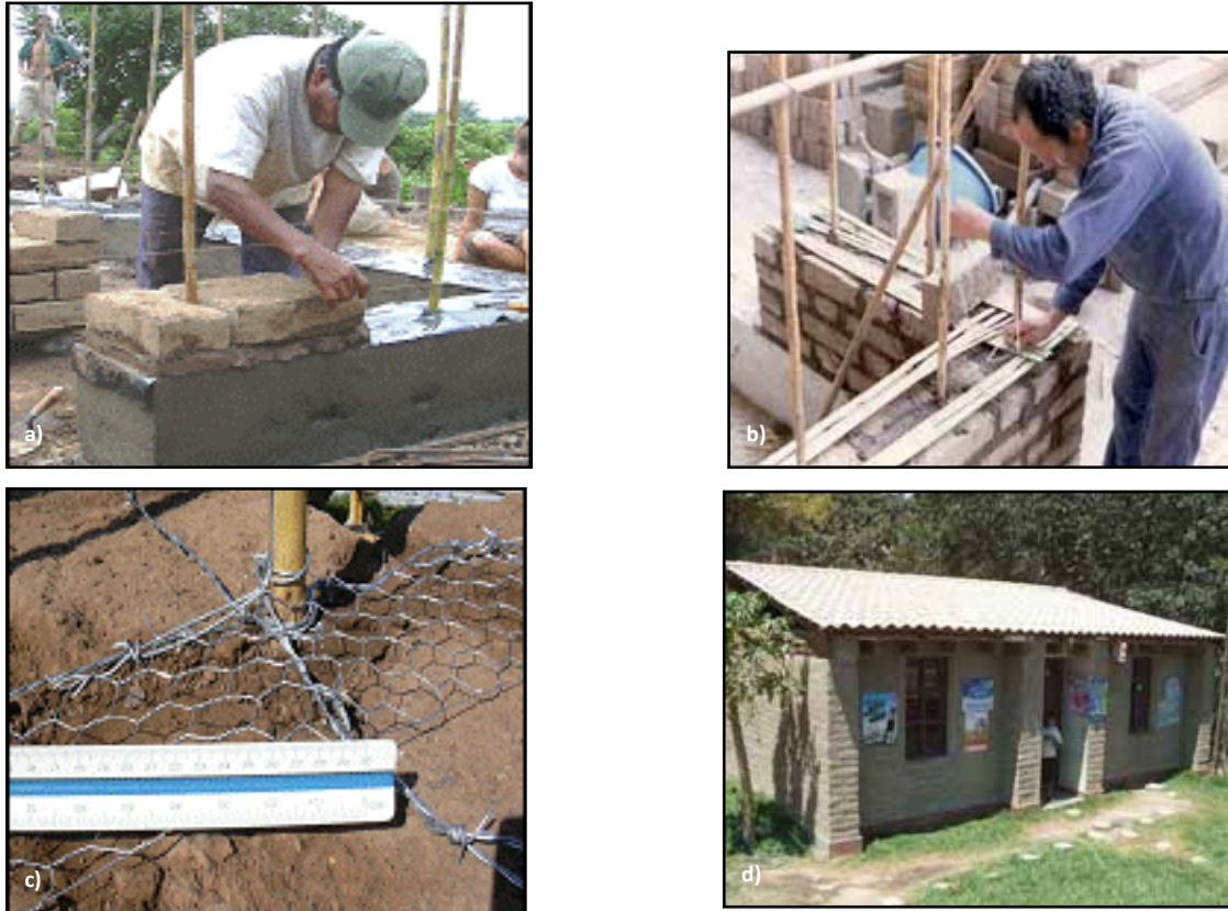
Figure 4.3 Construction with cane reinforcement in Peru and El Salvador: a) Placement of cane reinforcement, b) Vertical and horizontal reinforcement, c) Barbed wire as horizontal reinforcement, and d) House reinforced with cane and pilasters
