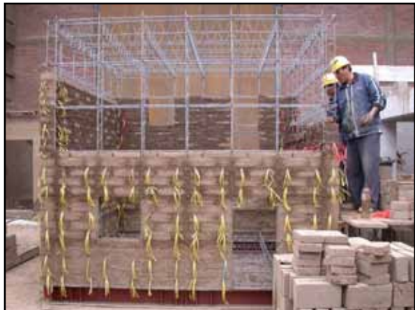
Figure 4.17 Construction of a building model using the integral masonry system
