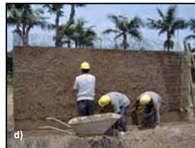
Figure 4.11 Construction details for the geomesh reinforcing scheme: a) Geomesh anchored to the foundation, b) Geomesh attached to adobe walls, c) Geomesh attached to the ring beam, and d) Geomesh covered with mud plaster
