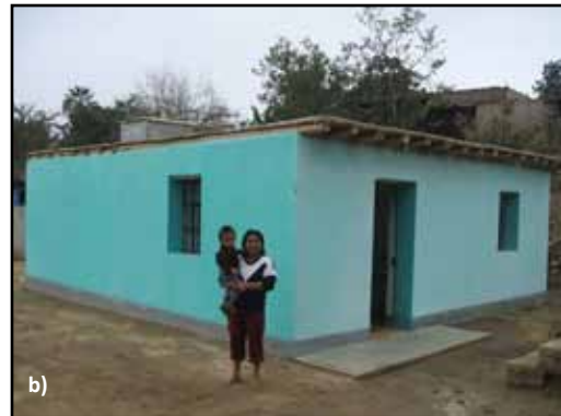
Figure 4.14 Reinforced adobe houses in Chincha, Peru built after the 2007 Pisco earthquake: a) A model house from PUCP-CARE's booklet, and b) Reinforced adobe house built by CARE
