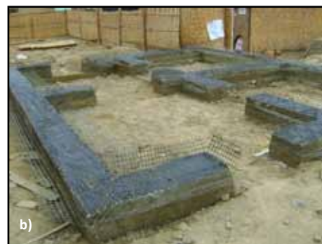
Figure 3.7 Protection of adobe walls against damp: a) Adobe walls with a concrete foundation, and b) Liquid asphalt on a foundation
