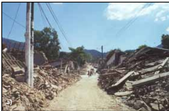
Figure 2.1 Collapsed adobe buildings: a) 2001 El Salvador earthquake (photo: D. Dowling), and b) 2003 Bam, Iran, earthquake (source: Mehraïn and Naeim 2004)
