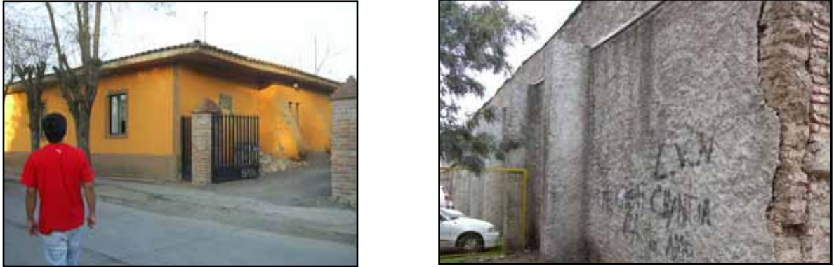
Figure 4.19 Adobe buildings with a buttresses and pilasters in Chile (photos: M. Moroni, S. Brzev)
