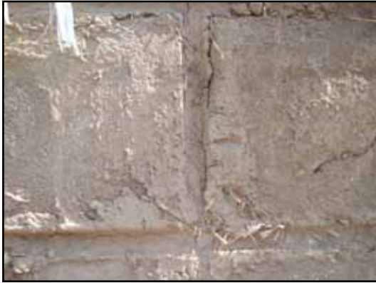
Figure 3.8 Mortar joints that are uniform and completely filled
