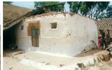
Figure 6A: Typical Earthquake Damage - Cracking and Separation of Walls in the 1997 Jabalpur Earthquake (Source: Sudhir K. Jain, IIT Kanpur)
