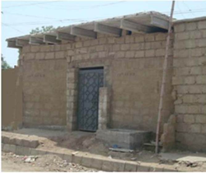
Figure 2. Concrete block masonry house, Karachi.
