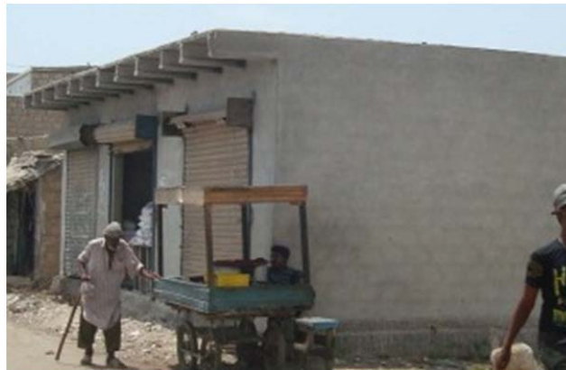
Figure 12. Block masonry with concrete girder roof and concrete tiles.
