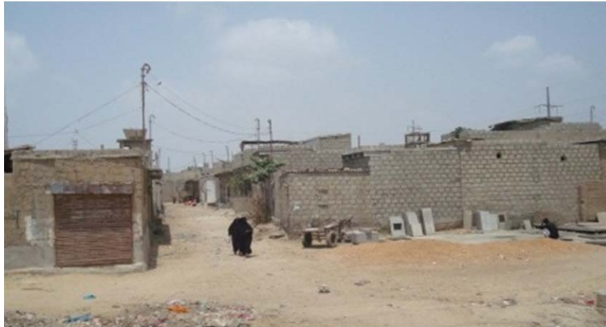
Figure 4. Typical block masonry settlement, Karachi.
