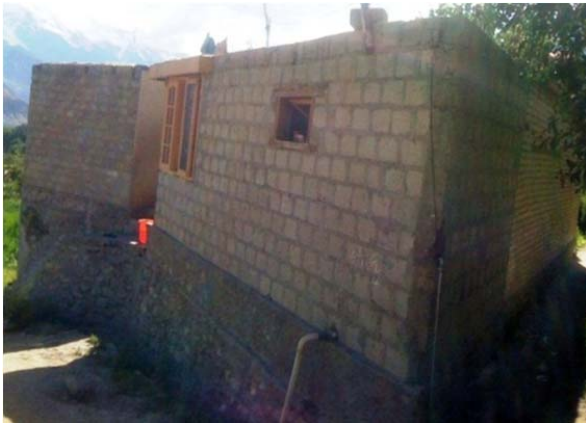
Figure 10. Stone plinth and foundation underneath block masonry.
