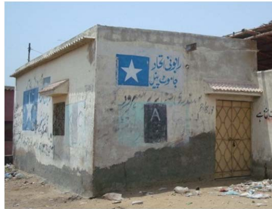
Figure 11. Block masonry with CGI sheet roof held down by a plastered parapet of blocks.
