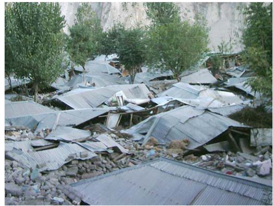
Figure 9. Collapse of unreinforced concrete block masonry houses in Kamsar near Muzaffarabad [5].
