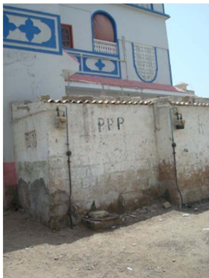
Figure 5. Adhoc appendage to the building.
