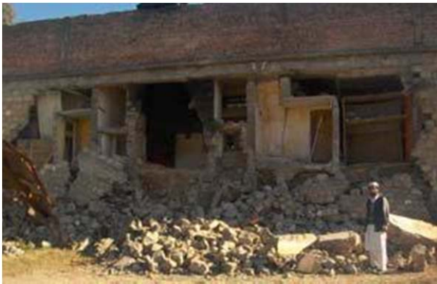
Figure 8. Out of plane flexural failure of load bearing wall constructed with block masonry in Kashmir Earthquake of 2005 [4].
