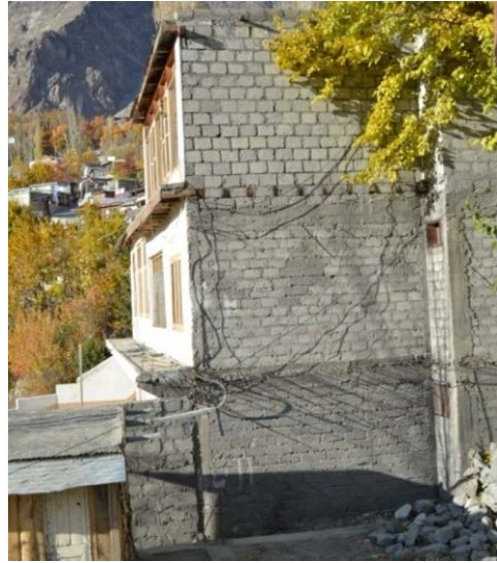
Figure 3. Concrete block masonry house, Northern Areas.
