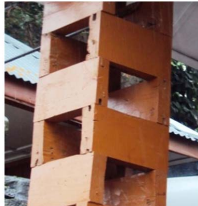
Figure 13. Connection principle of the Thola: (a) Joint detail of two Thatharas using wooden pins, (b) mortise and tenon joints.
