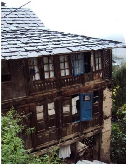
Figure 27. Change in roof angle over the verandah.
