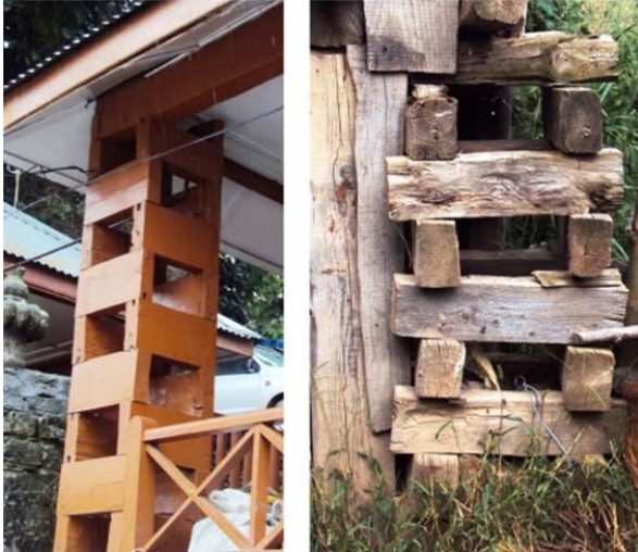
Figure 9. Hollow box-like frame (Thola) for Thathara construction.
