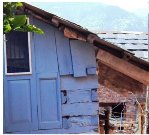
Figure 32. Slates nailed to purlins.
