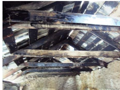
Figure 34. A-type roof frames.
