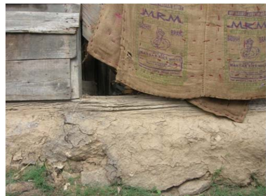
Figure 17. Stone foundation rising above ground level, in a typical Thathara house - village Rohta, Chamba district (Himachal Pradesh).
