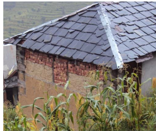
Figure 6. Bricks without mortar have been used to replace the worn-out portion of a wall.
