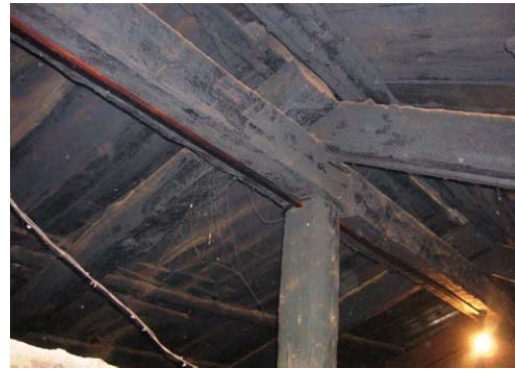
Figure 30. Main beam (Nhas) supported over intermediate wooden post (Thamb).
