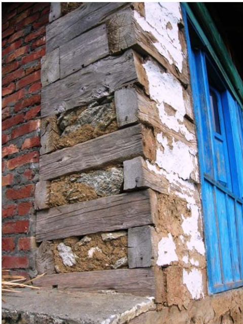
Figure 11. Thola with stone and planks laid together.
