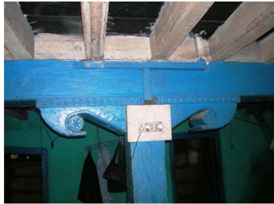
Figure 24. Main beam supported over the wooden post (Thamb) in the middle of the room.
