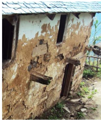
Figure 20. (a) Mud plastered exteriors of a Thathara house, (b) a mud plastered Thola.
