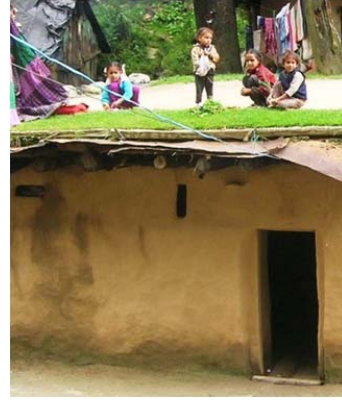
Figure 36. A flat roof unit.
