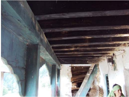
Figure 23. Main beam supported over the posts (Khambe) in the verandah and secondary beams also laid over the main beam.
