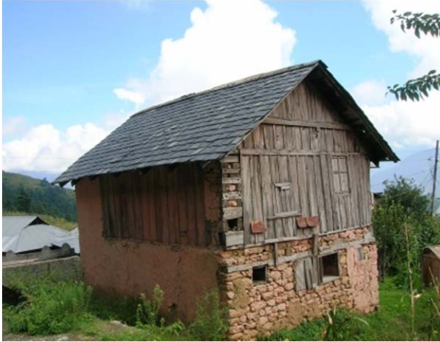
Figure 18. Thathara house with ground storey entirely made of stone.
