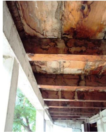
Figure 26. Planks laid over secondary beams.
