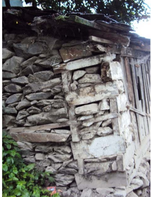
Figure 10. Thola with hand-packed stones.
