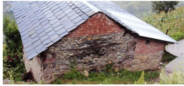
Figure 4. The combined use of dry stone masonry, stones with mud mortar and fired brick stones with cement mortar at a single house.
