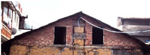
Figure 5. Fired brick stones with cement mortar have replaced earlier wall materials.
