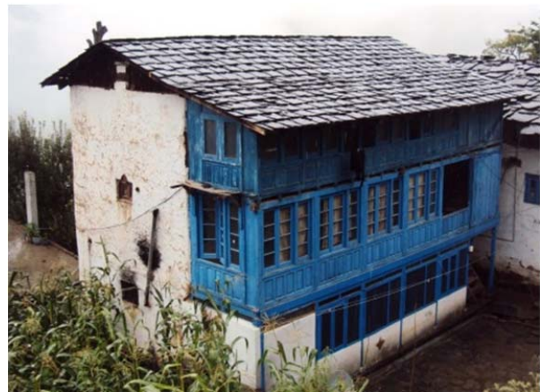
Figure 8. Verandah at ground floor has been enclosed by brick walls.
