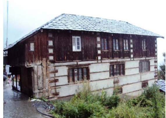
Figure 15. Wooden planks as infill in the upper storey - village Bharmour, Chamba district (H.P.).
