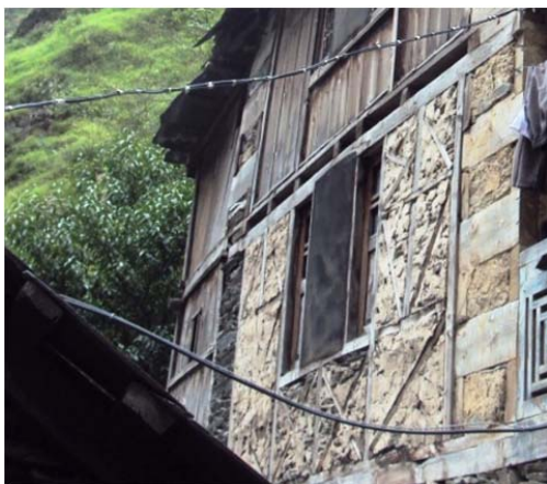
Figure 16. Dhajji-Dewari partitions, diagonal bracings made of wood.
