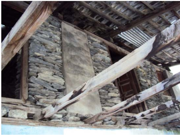
Figure 25. Stones filled in the gap between the secondary beams.
