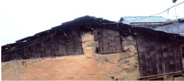
Figure 29. Main beam (Nhas) supported by the exterior column (Thola).
