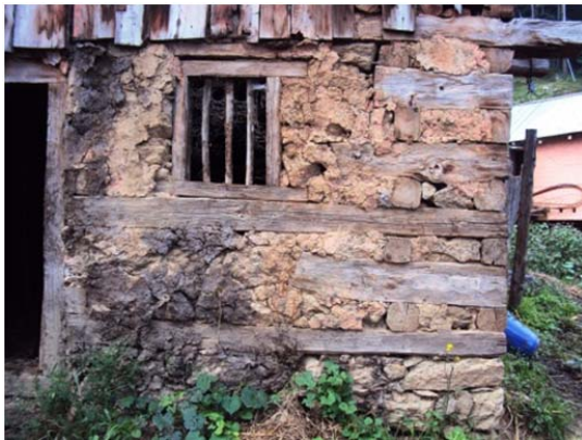
Figure 14. Stones with mud mortar as infill material.
