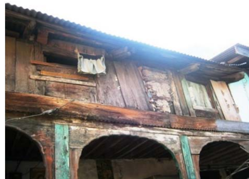
Figure 22. A house where the Thola can be seen above the wooden posts of the verandah.
