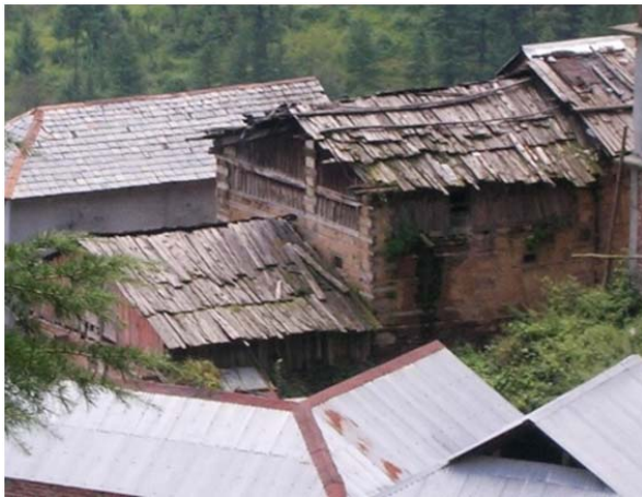
Figure 7. A Thathara house with the traditional roof covering type using wooden planks.
