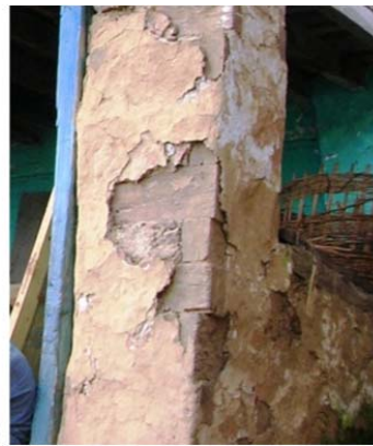
Figure 20. (a) Mud plastered exteriors of a Thathara house, (b) a mud plastered Thola.
