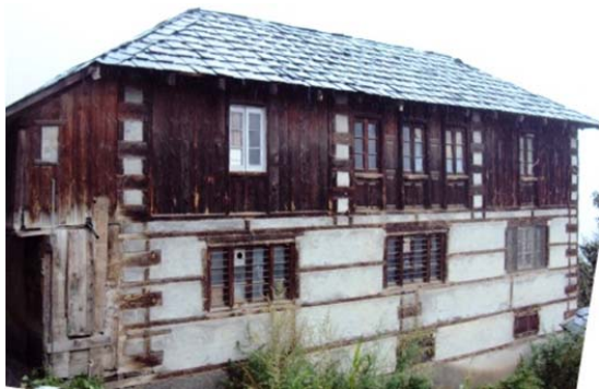
Figure 33. A Thathara house with hipped roof.
