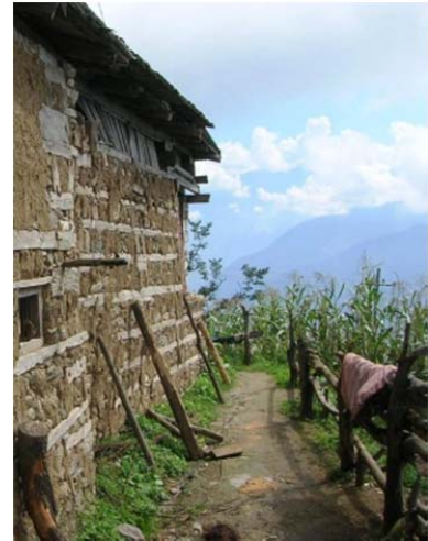
Figure 19. Horizontal wooden courses in between courses of stone.
