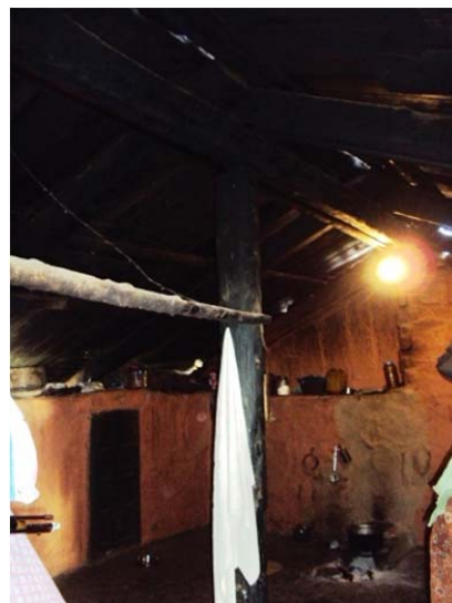
Figure 28. Gable end roof where ridge beam (Nhas) is supported over the Thamb in the center and the Thola at the gable end.
