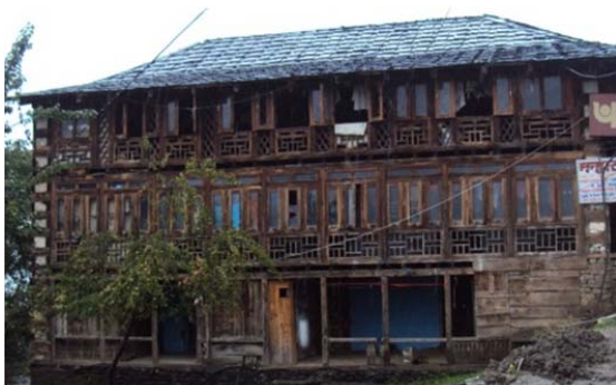
Figure 21. A house with verandah where walls in storeys above verandah are entirely in wood with large openings.
