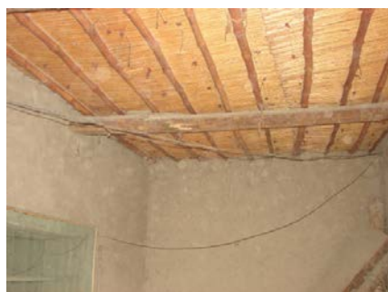
Figure 7: Adobe house roof - interior. Timber planks with bamboo stalks supporting wooden chick.
