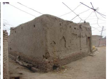
Figure 3: A typical adobe house, Larkana, Sindh.
