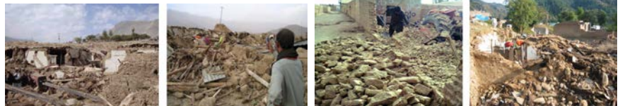
Figure 9: Total collapse of adobe houses during the Ziarat earthquake in 2008.
