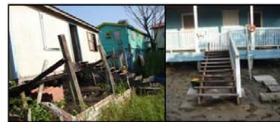
Figure 5: Stilt houses fell off their timber posts during the 2009 earthquake
