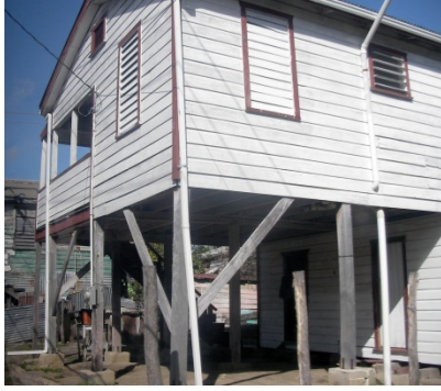
Figure 2: Typical wooden stilt home with a shed added underneath
