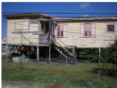
Figure 4: Wooden stilt houses may be poorly maintained, but still occupied
