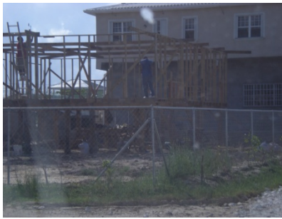
Figure 6: Construction of a timber stilt home
