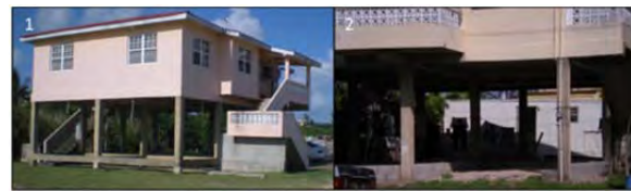
Figure 5: Typical building with (1) stilt construction and (2) later an infill wall being added at ground level.
