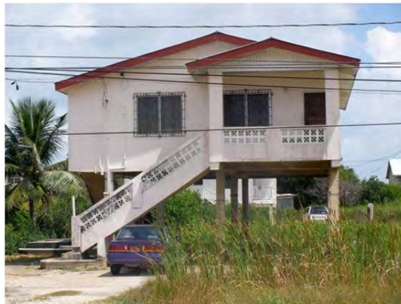
Figure 1: Typical concrete stilt frame home.
