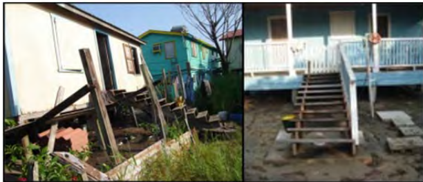
Figure 6: Damages observed after the 2009 earthquake: wood stilt buildings toppled, or sunk several feet into the ground.
