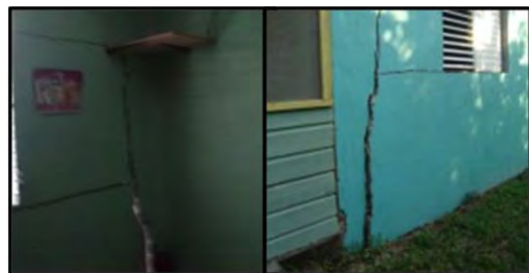
Figure 8: Cracking of masonry after the 2009 earthquake.
