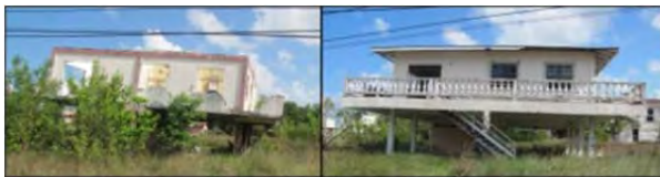
Figure 7: Highly variable soil conditions, these houses have been abandoned after sinking several feet.
