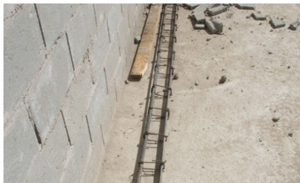
Rebar cage for RC ring beam
