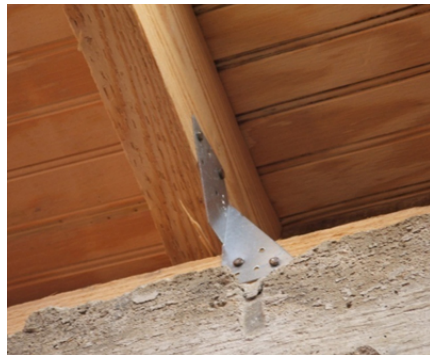
Timber roof beam to wall plate connection
