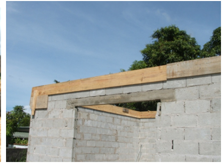
Formwork for RC ring beam
