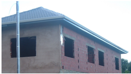
Photo of URM clay tile house
