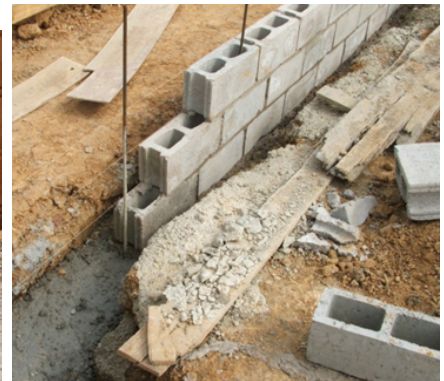
Stem wall of foundation for load-bearing walls
