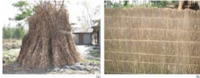
Figure 9: (a) Storage of Ikra reed for further use, and (b) making of Ikra roof and boundary wall.
