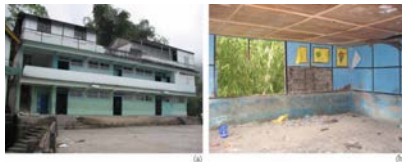
Figure 12: (a) Construction of additional Ikra type class rooms on third floor (on right side) of a reinforced concrete school building, and (b) damage sustained by the walls of the class rooms during 18 September 2011 Sikkim earthquake.
