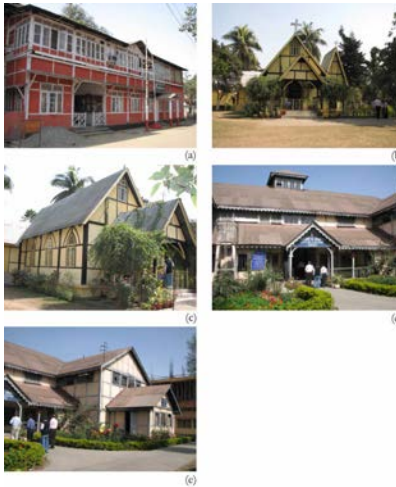
Figure 4: Changes in basic configuration of Assam-type houses as per the functional requirements: (a) a century old government Municipal Corporation building at Guwahati, (b) front view of Assam-type Church, (c) side view of Assam-type Church at Guwahati, (d) front view of Century Old single storey Cotton College Building, and (e) side view of Cotton College Building at Guwahati.
