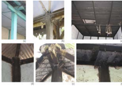
Figure 6: Connection between: (a) posts and horizontal rafters at verandah, (b) posts and horizontal rafters at eaves level, (c) post and ceiling, (d) post, rafters, and inclined roof member at eaves level from inside, (e) post, rafters, and inclined roof member at eaves level from outside, (f) post, rafters and asbestos sheet used for roofing.
