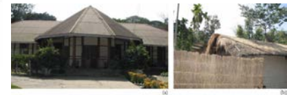
Figure 11: Commonly used roofing system: (a) CGI sheets, and (b) Ikra reed.
