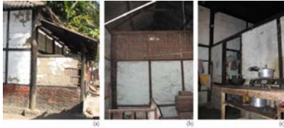
Figure 13: (a) Details of mud-dung plastering on walls, (b) and (c) arrangement of internal walls.
