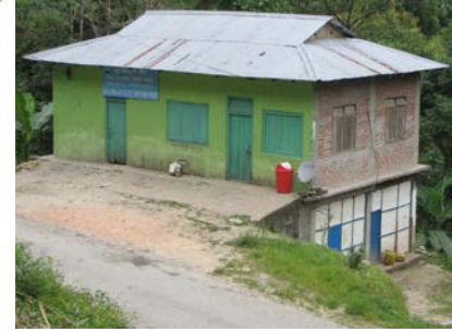
Figure 5: A vulnerable modification to the Ikra-type housing in Sikkim: heavy masonry infill walls above and light-weight Ikra walls below.
