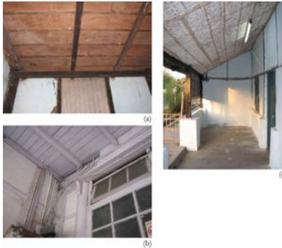
Figure 10: Variants of ceiling observed in typical Assam-type houses: (a), (b) wooden ceiling, and (c) ceiling made using Ikra reed and bamboo similar to roofs.
