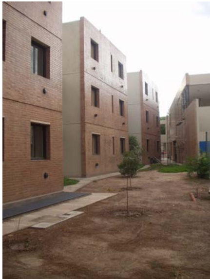
View of confined masonry buildings (North)
