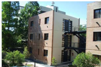
View of building with base seismic isolation
