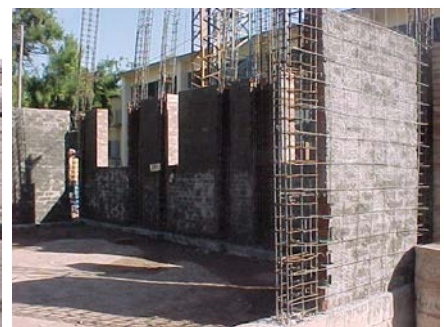
Details of Confined Masonry Walls. Note the layer of reinforcing mesh on the wall that will be covered with concrete in order to improve wall strength and ductility.
