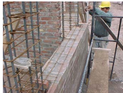
Construction of Reinforced Masonry
