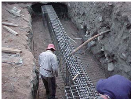
Construction of Reinforcement of Footings of BSI Building (B1x and B2X)
