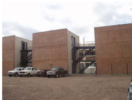
View of confined masonry buildings (South)
