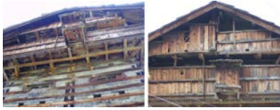
Figure 20. Toilet (outhouse) attached to the balcony at fourth floor at the buildings backside.
