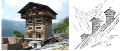
Figure 1. General view of a typical building located in Rajgarhi area and a sketch taken from Middlemiss (1910) illustrating structures of this type in the Kangra Valley.
