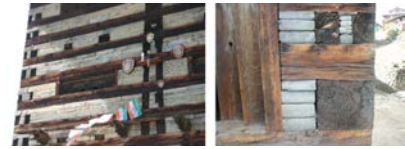
Figure 11. Arrangement of wooden logs and well-dressed flat stones for the walls.
