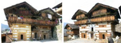
Figure 3. Representatives of Koti Banal structures being located close to each other.
