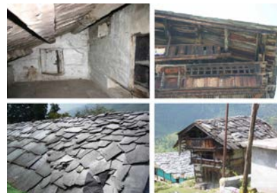
Figure 19. Detailing of the wooden roof construction and the roofing by large slate tiles.
