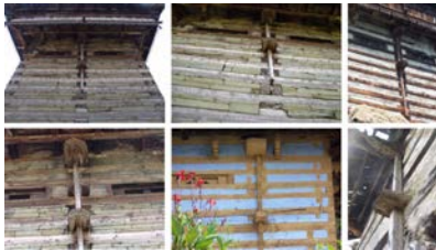
Vertical members ('shear keys') attached to the outer façade to prevent out-of-plane failure of the walls.
