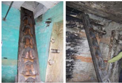
Figure 15. Ladders made of a single trunk used for access to upper floors.
