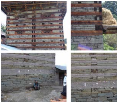
Figure 10. Arrangement of wooden logs and well-dressed flat stones for the walls.
