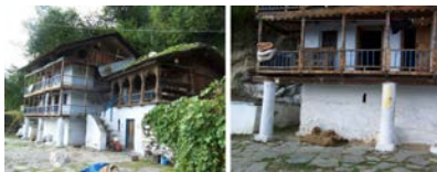
Figure 16. Modification of the Koti Banal construction principle: arrangement of external verandas resting on massive columns.
