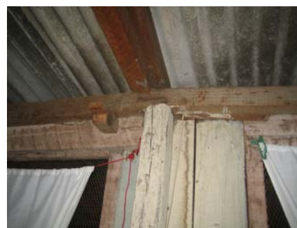
Figure 7: Roof made of asbestos sheets supported by wooden beams
