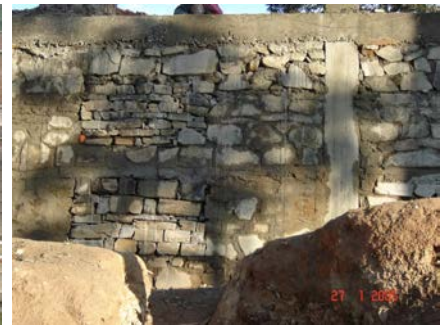
Infill wall in stone masonry
