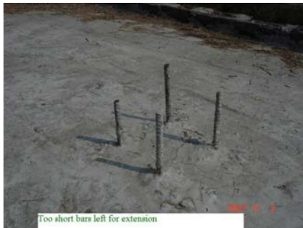
Too short bars left for extension Column reinforcement is far too short for the continuity of the column
