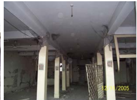
Onset of plastic hinging at top of columns
