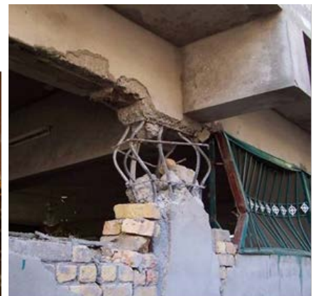
Short column due to partial height infill wall
