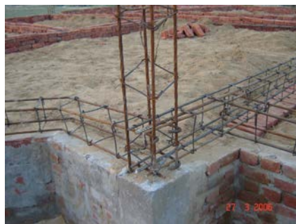
Beam reinforcement hooking into column reinforcement. Also note inadequately large spacing of stirrups in the beam and column, and no stirrups in beam-column joint.
