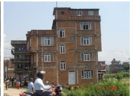
Missing beams
