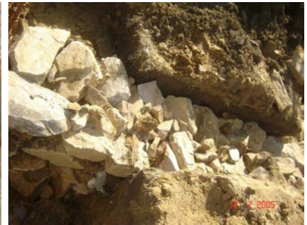
Constructing toe wall for tie (at plinth level) beam in stone masonry
