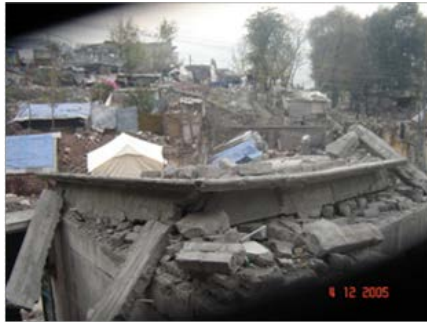
Deficient lap length, and very poor lap location leading to partial collapse of the building
