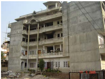
A typical RC frame building with masonry infill
