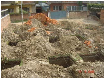
Pits for isolated footings
