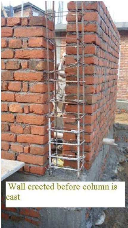
Infill wall erected before concreting column
