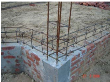
No anchorage of beam bars in column
