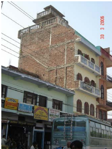
Column starting from 5th storey
