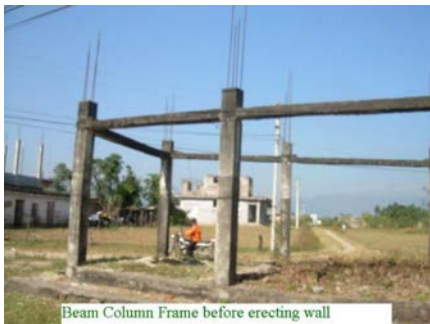
RC frame ready to receive infill walls. Note that there are no horizontal ties protruding from the columns to prevent the infills from falling out of the frame.
