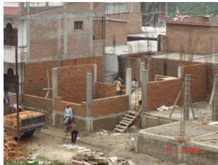
Infill wall under construction
