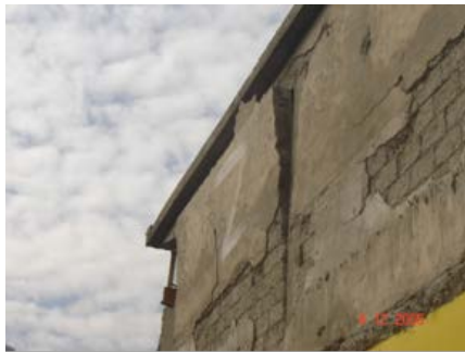
Onset of out-of-plane collapse of infill wall
