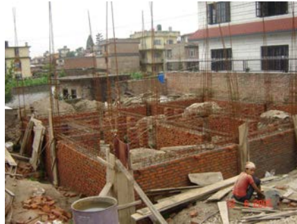
Plinth/ tie beam construction
