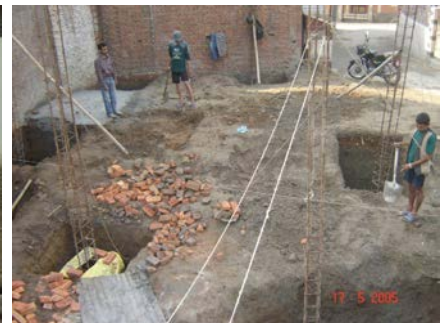
Isolated footings under construction
