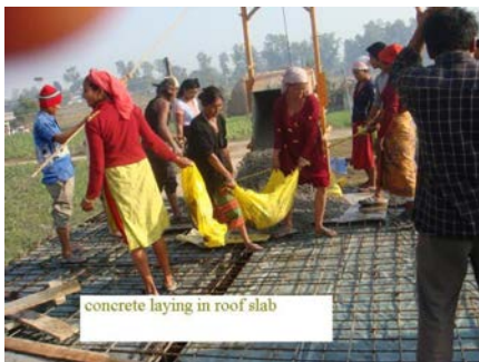
Construction of floor slab
