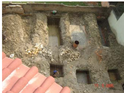
Pits for combined foundation
