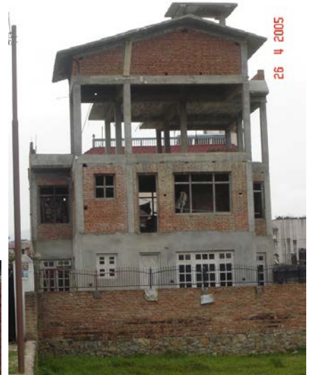
Building with bottom storey ineffectively infilled because there are no solid bracing panels. The top storey is infilled and all the storeys below are very weak and vulnerable.
