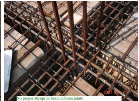
No proper stirrups in beam-column joints No stirrups in beam-column joint
