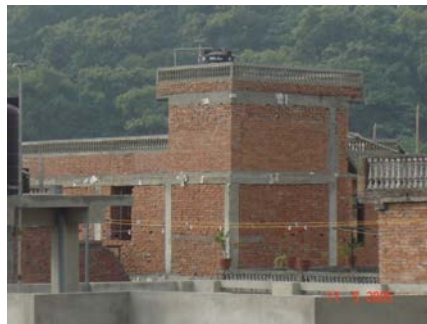
Missing columns in top storey
