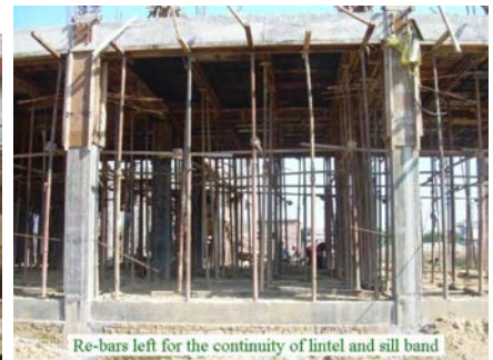
RC frame under construction (note anchor bars at lintel and sill level for respective bands to tie the infill walls)
