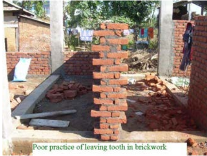
Tooth in brick work for extension of walls
