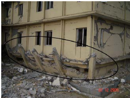
Shear failure of first storey columns
