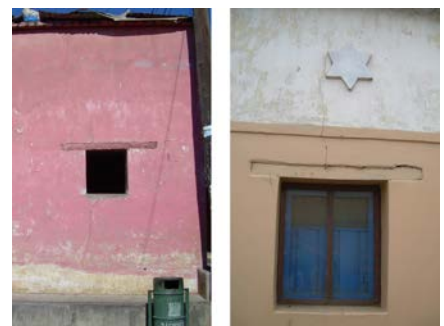
Figure 6. Window lintels consisting of wooden trusses.
