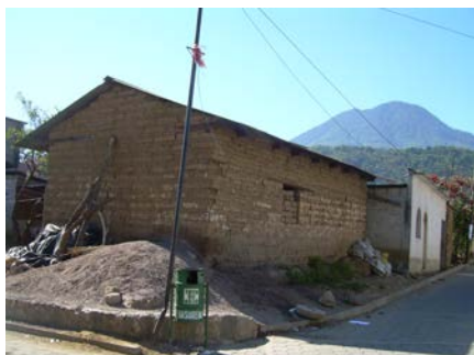
Figure 1. Typical adobe building for rural areas (San Juan La Laguna). [Click to enlarge figures]
