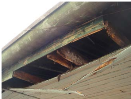
Figure 9. Rotten beams of the wooden roof construction.
