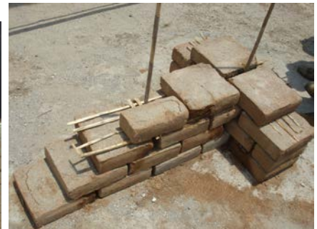
Figure 10. Principle of internal wall reinforcement with bamboo (Universidad de El Salvador UES, 2007).
