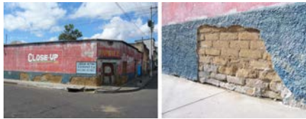
Figure 8. Spalling of plaster due to ascending moisture in the adobe walls (Guatemala City, Zona 7). [Click to enlarge figures]
