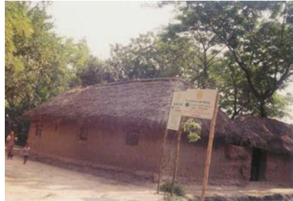
Figure 12: Mud house with straw roof
