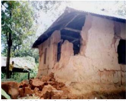
Figure 25. Collapse of mud house due to the 2003 Barkal earthquake (EERC, CUET)
