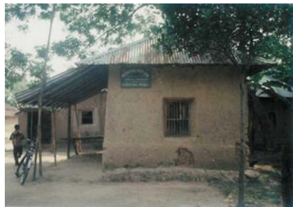
Figure 15: Mud house with corrugated galvanized iron sheet roof
