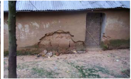
Figure 27. Typical damage at a mud house in Hathazari, Chittagong (Iftekhar, 2007)
