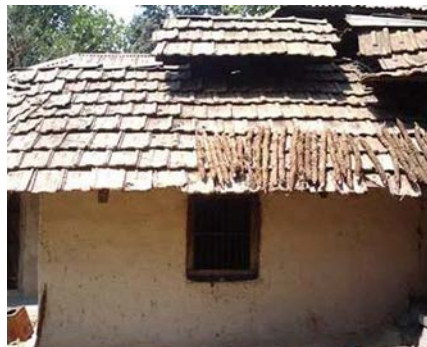
Figure 18. A building with tile roof supported by wooden purlins in Pahartoli, Raozan, Chittagong (Rebeka Ahsan, 2006; Firoza Akter, 2007)
