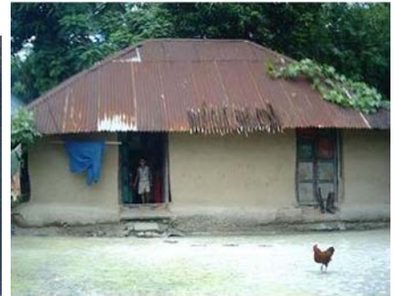
Figure 13. CI sheet roof supported by wooden purlins (Firoza Akter, 2007)
