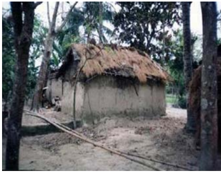
Figure 11. A building with thatch roof supported by wooden purlins in Muktagacha, Mymensingh (Asraful Aslam, 2006; Firoza Akter, 2007)
