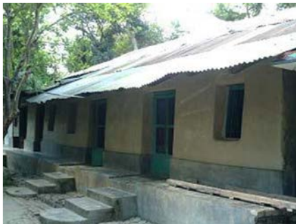
Figure 17. Too many openings provided in one wall (Firoza Akter, 2007)
