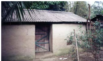
Figure 1. Typical building with tin roof in Muktagacha, Mymensingh (Asrafal Alam, 2006)
