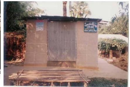
Figure 19. Mud house with flat roof supported by bamboo joists
