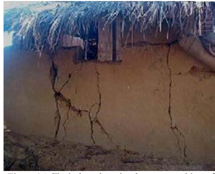
Figure 26. Typical earthquake damage: cracking of walls due to the 2003 Barkal earthquake
