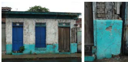
Figure 14. Bahareque building in an urban area with a pedestal made of clay bricks.
