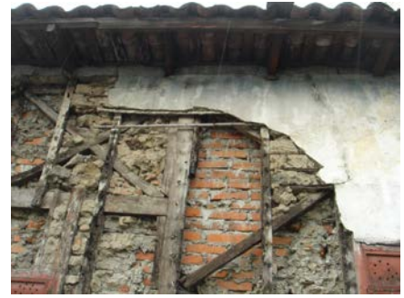
Figure 10. Modification of a bahareque house by an additional wall at the inside made of masonry bricks (Santa Tecla).
