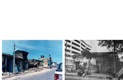
Figure 17. Damaged bahareque dwellings after the San Salvador earthquake on October 10, 1986 (left: San Jacinto neighborhood; right: after Kuroiwa, 1987). [Click to enlarge figures].
