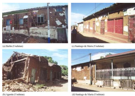
Figure 18. Structural damage to bahareque dwellings caused by the earthquake on January 13, 2001.
