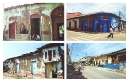
Figure 19. Structural damage to bahareque dwellings in the city of San Vicente caused by the earthquake on February 13, 2001.
