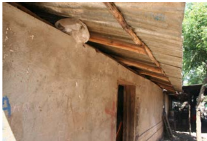
Figure 8: Timber roof framing and plastered wall.
