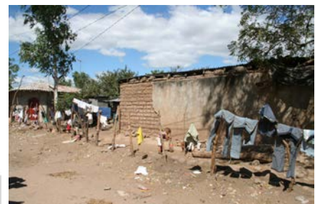
Figure 6: View from the road. The exterior plaster on the left side has fallen off due to the lack of eaves.
