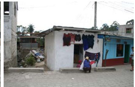
Figure 3: Front view of building from road.
