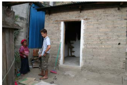
Figure 2: Rear view of building.
