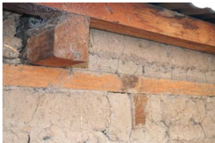
Figure 1: Connection of roof framing to wall incorporating a timber ring beam.
