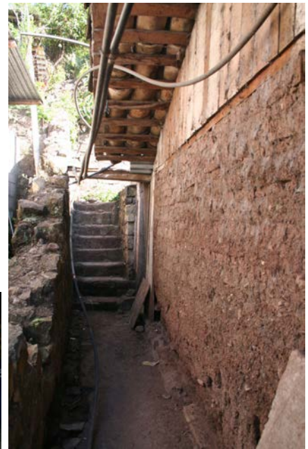
Figure 12: Side wall showing timber boards above wall and the weathering of the wall due to lack of plaster cover.
