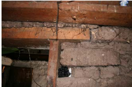
Figure 10: Lintel and wall connection.
