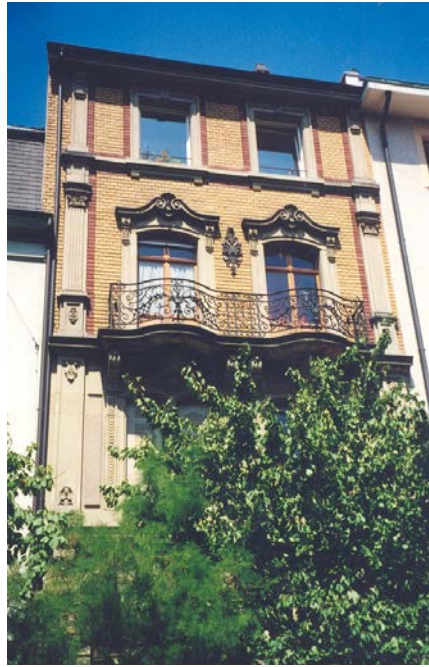
Figure 1b: Typical Building
