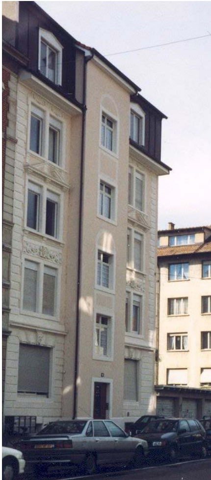
Figure 1a: Typical Building
