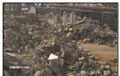
Figure 6 (d): Debris of buildings collapsed due to lateral thrust in addition to seismic forces. Note a building in the background with rigid diaphragm is still standing; Pakistan earthquake of October 08, 2005.
