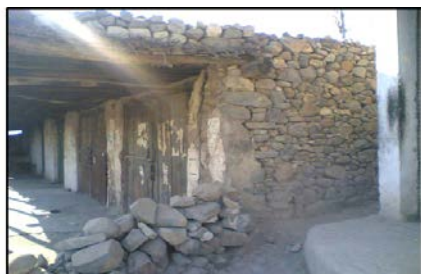
Figure 1 (a): A view of typical stone masonry house constructed in dry (without any mortar) with earthen roof.
