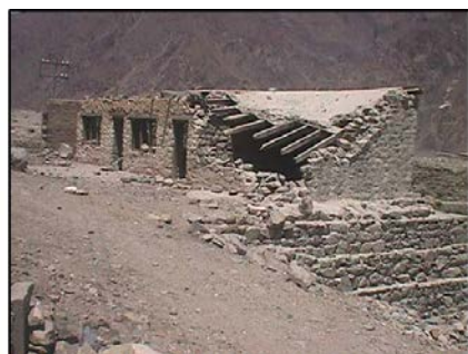
Figure 6 (a): Typical corner failure of a stone masonry house in mud mortar with earthen roof; Pakistan earthquake of October 08, 2005.
