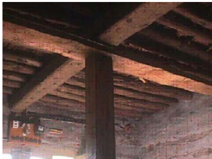
Figure 7: A wooden column in the center of a room, in addition to the main stone masonry walls, is provided to support roof gravity load
