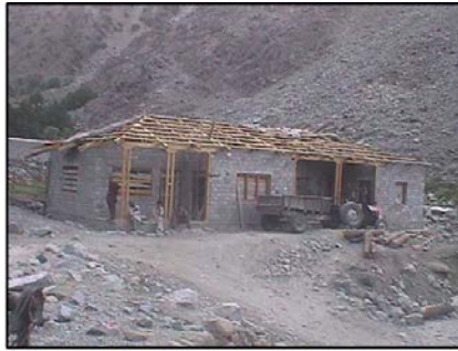
Figure 1 (f). A view of under construction stone masonry house in cement sand mortar with wooden truss and G.I. Sheet roof.
