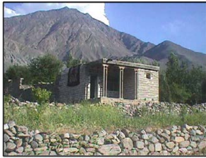
Figure 1 (d). A view of typical stone masonry house constructed in cement sand mortar with earthen roof.
