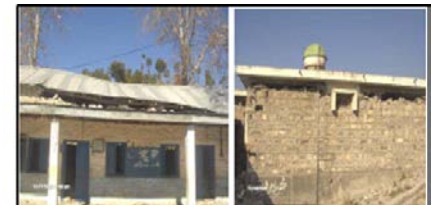
Figure 6 (f): Slippage of top course of masonry; Pakistan earthquake of October 08, 2005.
