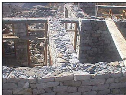
Figure 1 (b): A view of under construction stone masonry house in dry.
