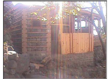
Figure 5 (e): An under construction house, being built with wooden seismic bands.
