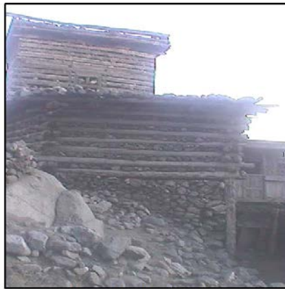
Figure 5 (a): An old house with wooden seismic bands.
