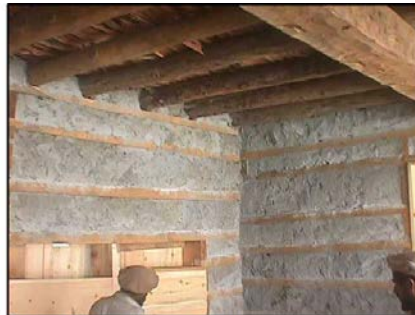
Figure 5 (d): Inner close view of building in fig 5 c.
