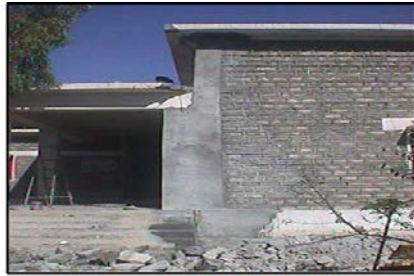
Figure 25: Seismic strengthening technique; column repaired after the earthquake
