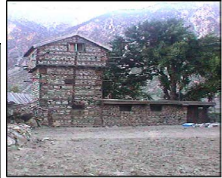
Figure 27: Seismic strengthening techniques; horizontal and vertical wooden bands introduced after the earthquake
