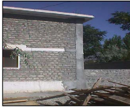
Figure 26: Seismic strengthening techniques; column repaired after the earthquake
