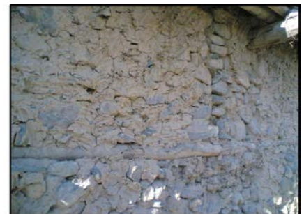
Figure 1 (c): A view of typical stone masonry wall constructed in mud mortar.
