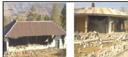
Figure 6 (e): Out of plane bending failure of masonry walls due to additional thrust from roof trusses; Pakistan earthquake of October 08, 2005.
