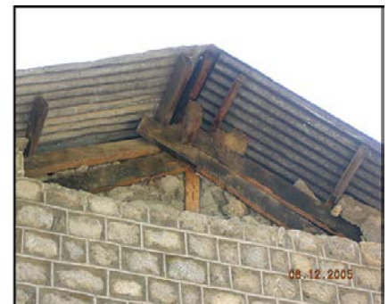
Figure 6 (c): Gable wall failure; Pakistan earthquake of October 08, 2005.
