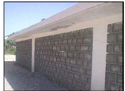
Figure 1 (g). A view of stone masonry house constructed with dressed stones in cement sand mortar having R.C.C. roof.
