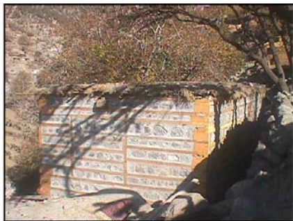
Figure 5 (c): A recently built stone masonry house in cement sand mortar and earthen roof; horizontal and vertical wooden bands are clearly visible.
