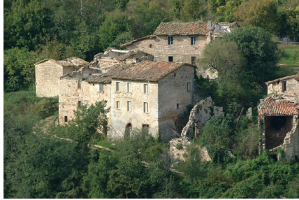
Figure 2: UMI 11 Le Cese overall view of the downhill elevation. The roof structure on the far side of the building (over the older portion) has completely collapsed.
