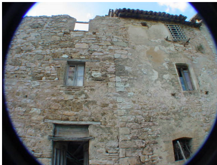
Figure 4: UMI 11 Le Cese view of the downhill exterior facade
