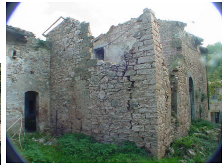
Figure 3: UMI 11 Le Cese view from the uphill side, where there are only two stories above grade. The residence sustained major damage to the stone masonry walls on this elevation in the 1997 Umbria-Marche earthquake. The roof completely collapsed as well.
