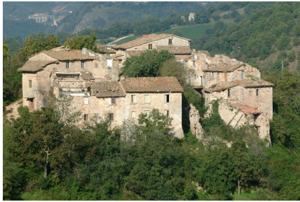
Figure 1: UMI 11 Le Cese overall view of the downhill elevation. UMI 11 is the structure immediately facing the hillside to the left of the photo. UMI 9, to the right of UMI 11, almost completely collapsed in the 1997 Umbria-Marche earthquake.
