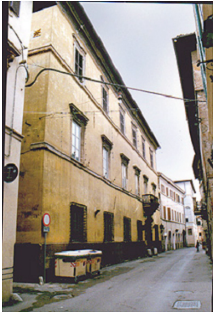
Figure 1: Front elevation view from street of upper class residential building, Palazzo Spinola, in Foligno, Umbria (Photo).
