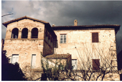
Figure 2: Exterior elevation view from street of the Palazzo Spinola in Foligno, Umbria (Photo).
