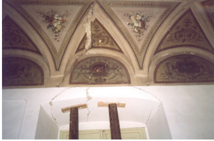
Figure 10: Damage to vaulted entryway and fresco ceiling detailing after the 1977 Umbria-Marche earthquake.
