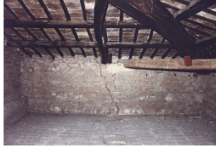
Figure 11: Cracked stone masonry wall at the top level of the residence after the 1977 Umbria-Marche earthquake.
