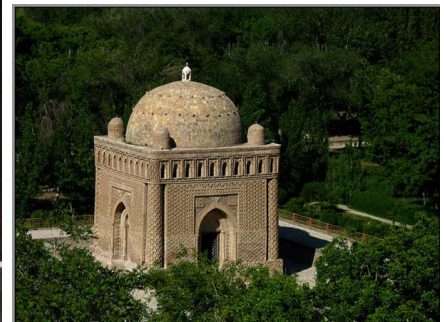
Figure 15: A Samanian king's house in Bukhara
