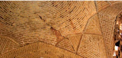
Figure 6: 1- Cracks in the dome-roof (it may not
