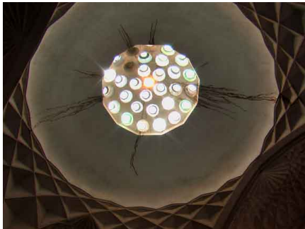
Figure 10: Roof opening for natural light because of lack of electricity in the past . This is the Ganjali khan bath in the city of Kerman.
