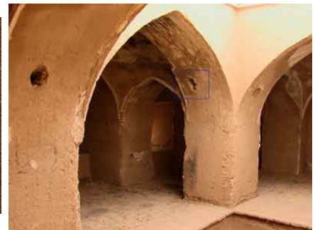
Figure 12: The holes that carry the timber tie beams to prevent slipping the roof. This building is located in the city of Aqda, province of Yazd.
