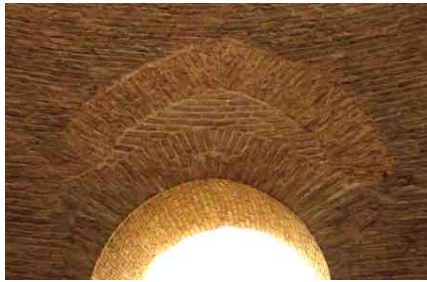
Figure 11: Modification and strengthening technique of arches. This is the Toqrol Tower, built around 400 A.D., in the city of Ray, province of Tehran.
