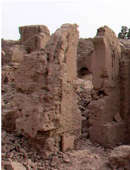
Figure 7: 2- Vertical crack on thick column (pier). This is from a structure built around 0 A.D. in the city of Bam, province of Kerman.
