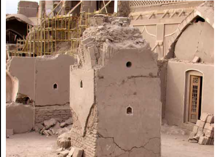
Figure 9: An Illustration of Key Seismic Features and/or Deficiencies. This is a building built around 0 A.D. in the city of Bam, province of Kerman.
